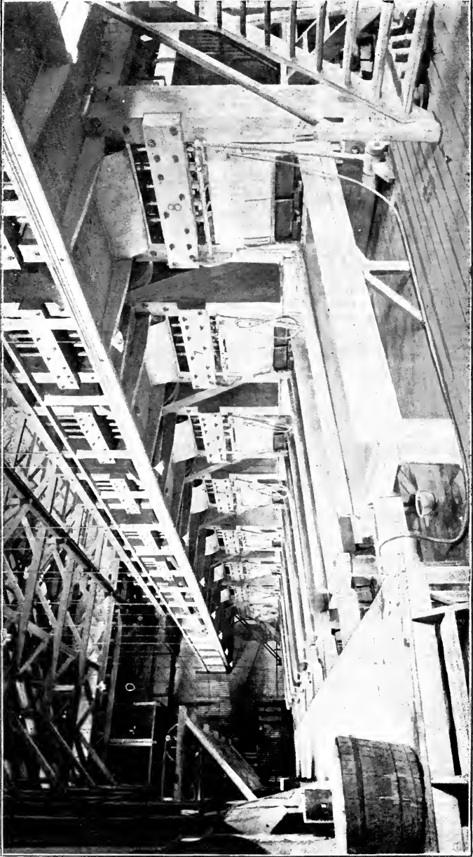
The 40-Stamp Battery of the New Heriot Company, showing the Stamps, Water-Supply, and Copper Tables. To face p. 220.
