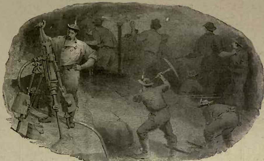
INGERSOLL DRILLS AT WORK IN THE NEW YORK AQUEDUCT TUNNEL.
