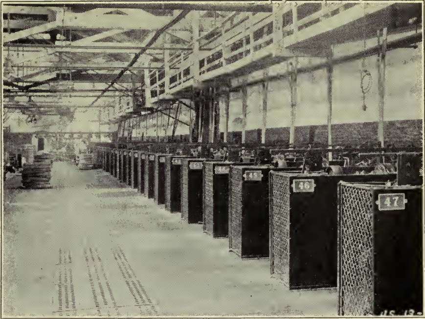
A row of barbed-wire machines, inclosed for safety
