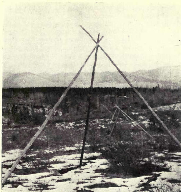
Fig. 19 Tripod line supports
