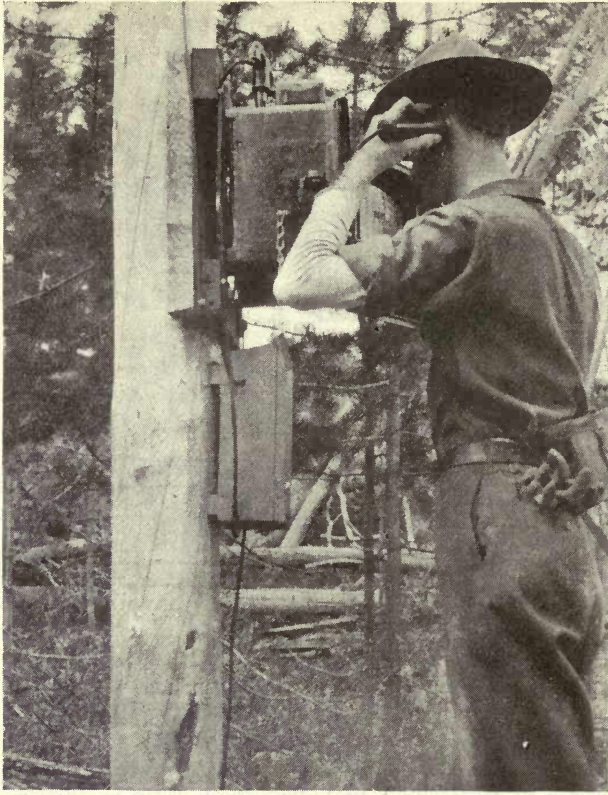
Fig. 48 Lookout station telephone set installed in the field
