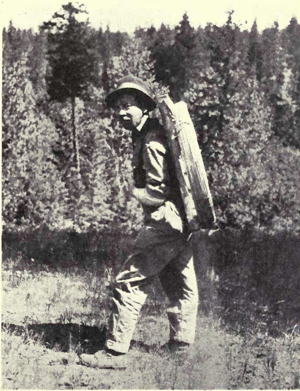
Fig. 8 Klondike pack-frame as used for packing wire
