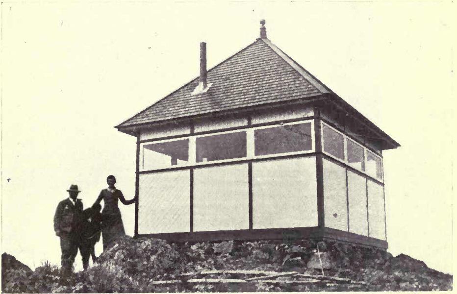
Fig. 1 Lookout station on a Dominion forest reserve in British Columbia
