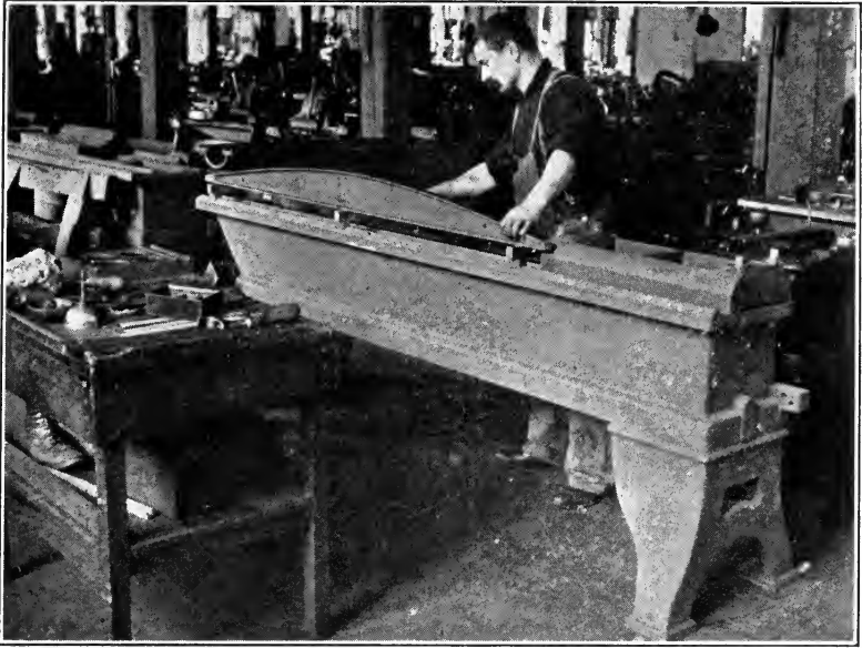
FIG. 10.—Testing a lathe bed for straightness.
