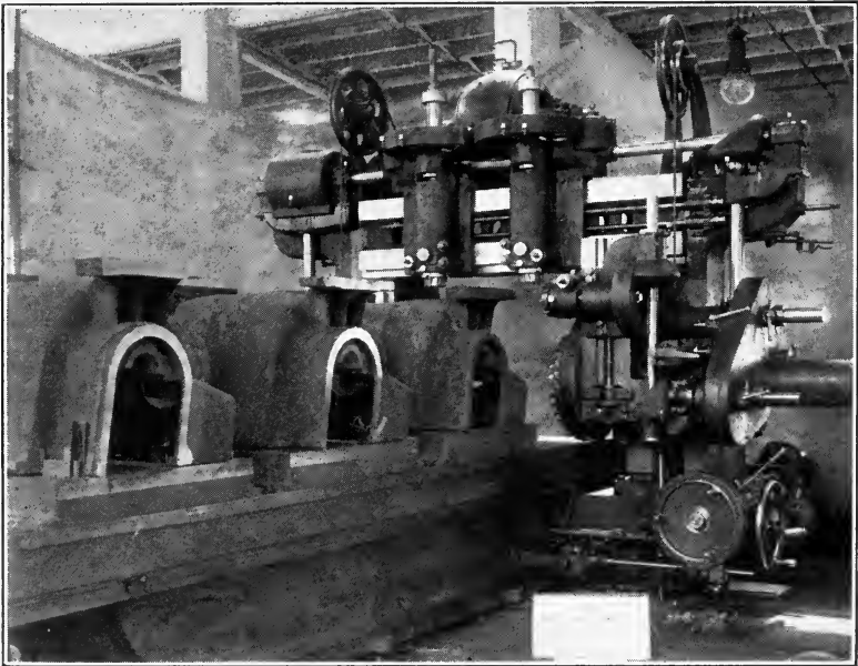
FIG. 218.—Multiple spindle planer type milling machine.
