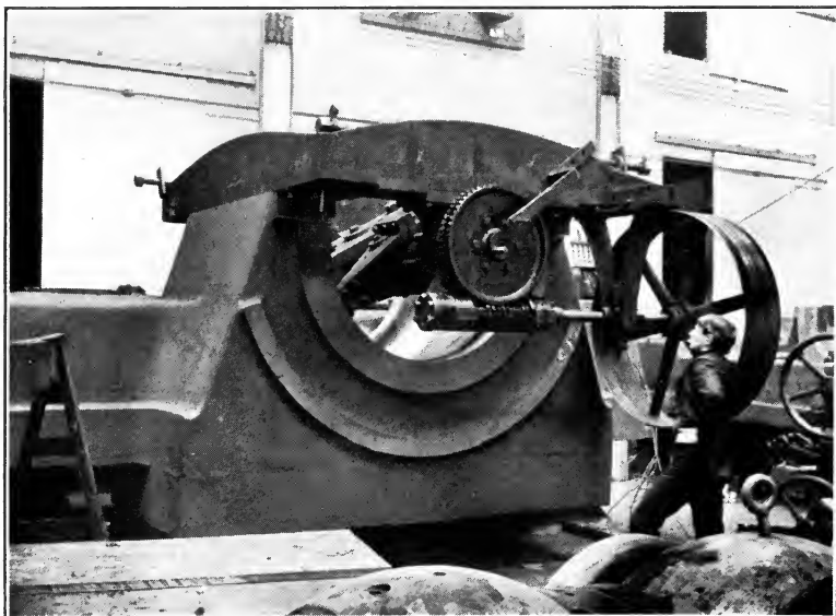
FIG. 168.—Boring spherical seats for bearings.
