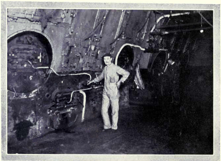
“SAN FRATERNO” OIL-FIRED FURNACES.
