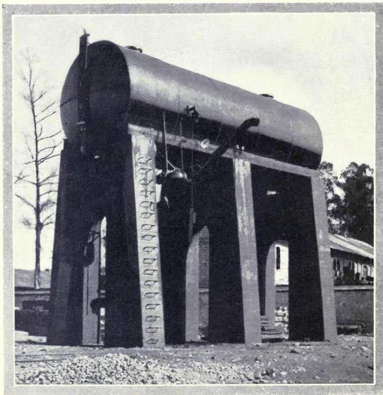
20,000-GALLON FUEL OIL TANK ON MEXICAN RAILWAY.
