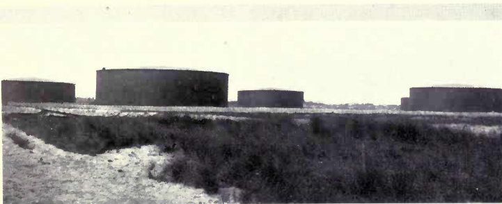
SOME OF THE 55,000 BARREL STORAGE TANKS, MEXICAN EAGLE OIL CO.
