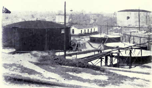
DISTILLATE RECEIVING TANKS, MINATITLAN.
