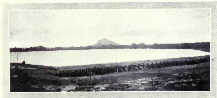
STORAGE RESERVOIR AT POTRERO—2,500,000 BARRELS.
