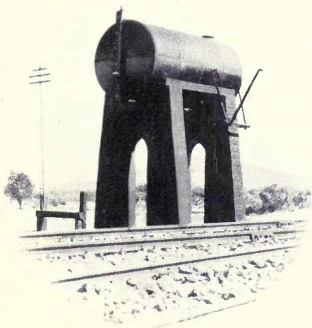
FUEL OIL SERVICE TANK ON MEXICAN RAILWAY.
