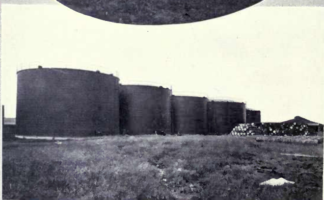
STORAGE TANKS AT BARTON, MANCHESTER.
