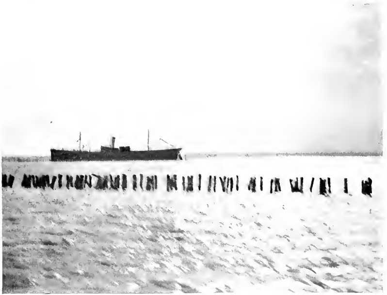
Piles showing all that remained of one of the four railway bridges washed away.
