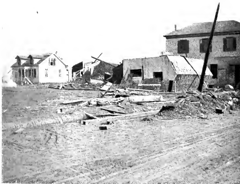
House blown over by the storm.
