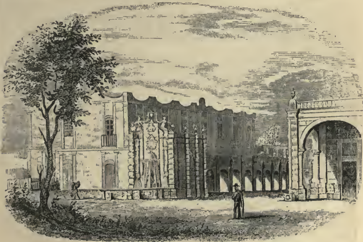
TERMINATION OF AQUEDUCT IN CITY OF MEXICO.
