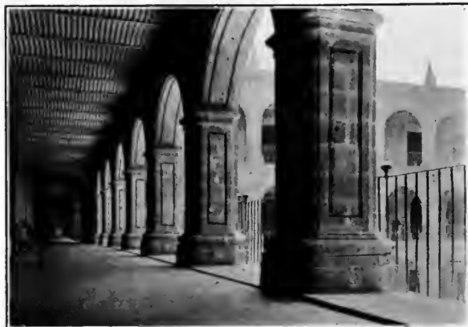
ENTRANCE TO SCHOOL OF ENGINEERS.
