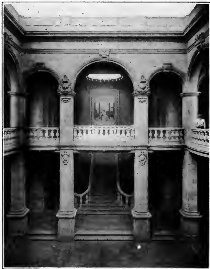
STAIRWAY IN THE INSTITUTE OF ARTS AND SCIENCE.
