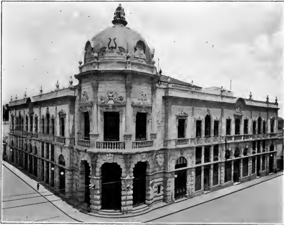
FAÇADE OF THE CASINO.
