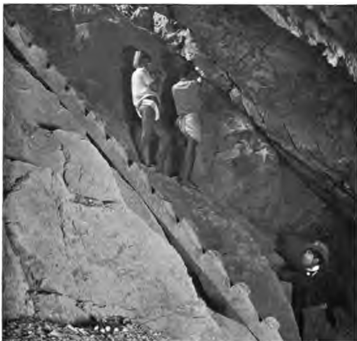
PRIMITIVE FORMS OF MINING.—Raising ore by the chicken-ladder.
