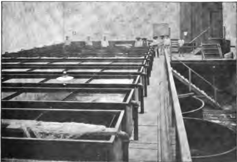
GUANAJUATO REDUCTION AND MINES CO.—Precipitating Plant.
