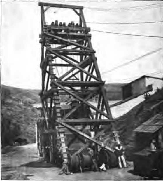
GUANAJUATO MINE.—Shaft and Electric Hoist at the Nuéva Luz Mine.
