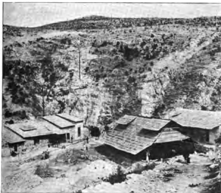
GUANAJUATO.—ENTRANCE TO THE PENGUICO TUNNEL.
