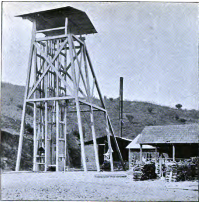
OAXACA MINES.—Gallows frame on the Vichache Mine, Taviche.
