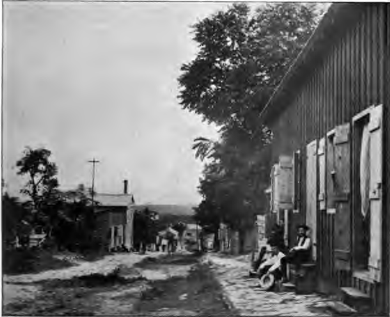
STATE OF TAMAULIPAS. A STREET IN TAMPICO.
