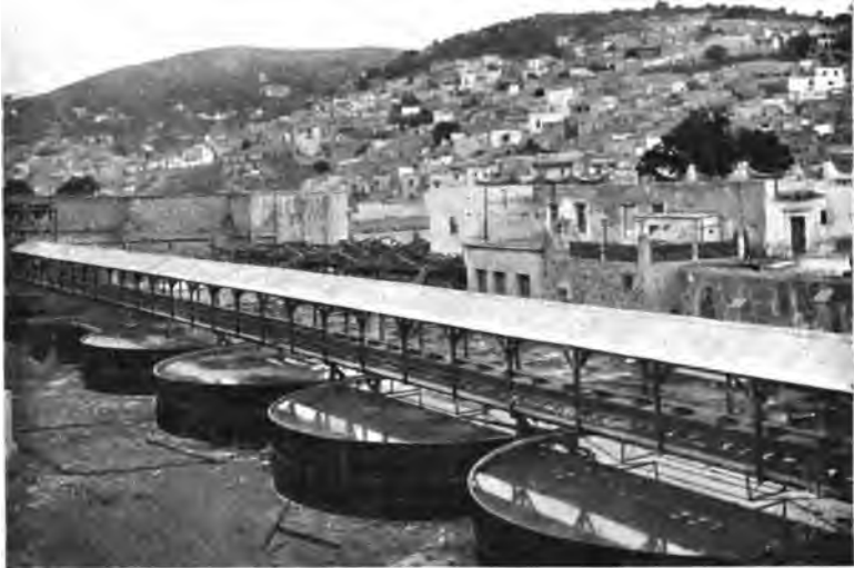
GUANAJUATO REDUCTION AND MINES CO.—Sand leaching tanks.
