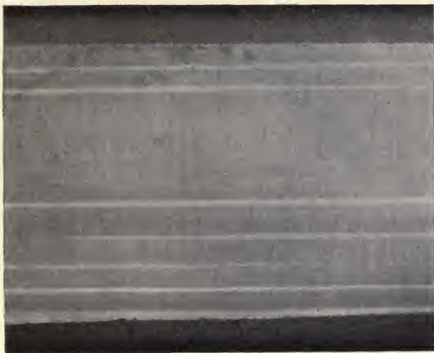
PHOTOGRAPH NO. 26. Light streaks in steel rail.
