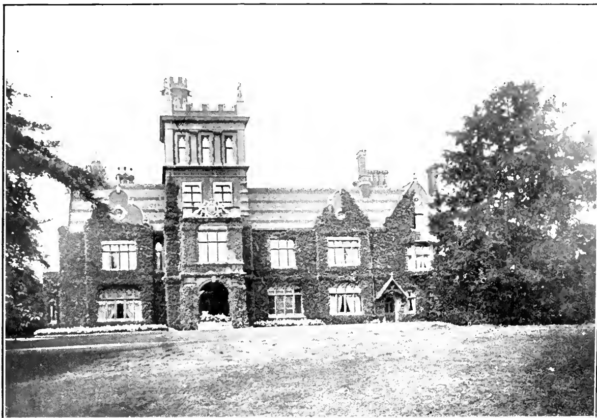
CAEN WOOD TOWERS (East View).
