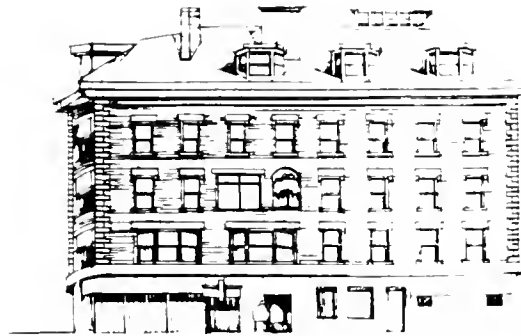
LIBERTY TREE BUILDING
