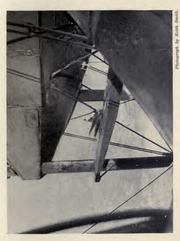
The hawk's wing jammed on one of the engine bracing wires.
