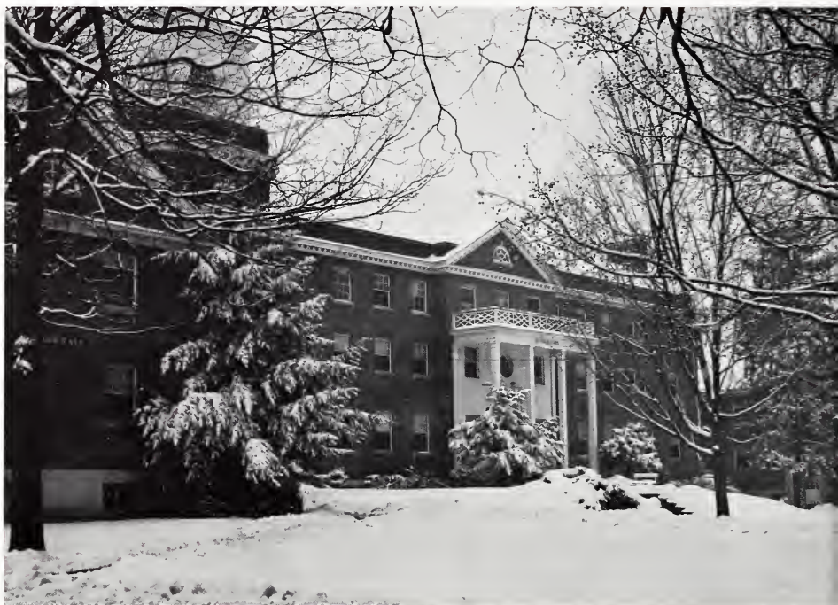
Above: Beckham Hall, one of five men's dormitories, stands at the entrance of Campus Drive.
