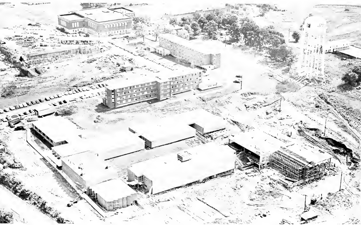
THE DONOVAN BUILDING is pictured nearing completion in this aerial photo, looking toward the growing Eastern campus from Lancaster Road.
