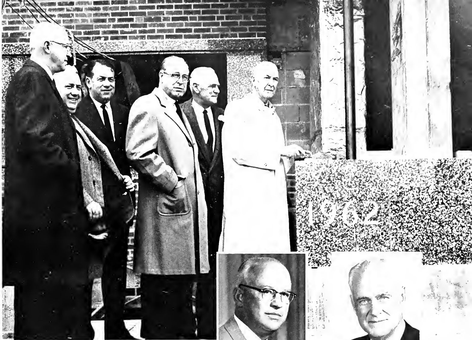
JUDGE THOMAS B. MCGREGOR is joined by other members of the College Board of Regents in laying the cornerstone for six-story McGreggor Hall, residence hall for women.
