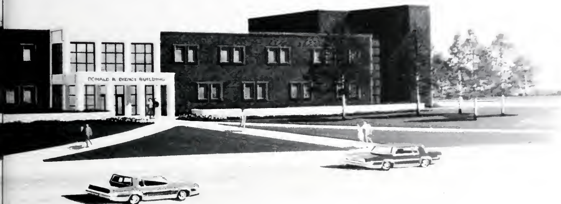
DONALD R. DIZNEY BUILDING COLLEGE OF ALLIED HEALTH AND NURSING EASTERN KENTUCKY UNIVERSITY Sherman · Carter · Barnhart Partners in Architecture
