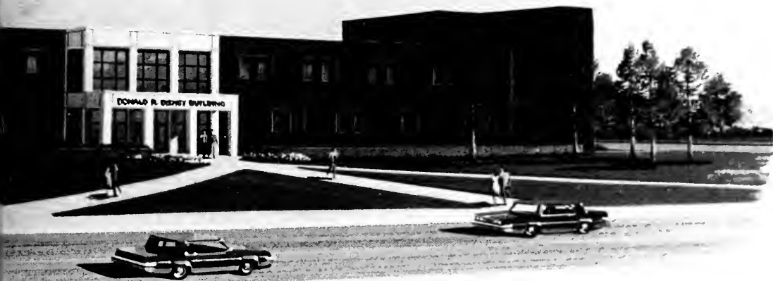
DONALD R. DISNEY BUILDING COLLEGE OF ALLIED HEALTH AND NURSING EASTERN KENTUCKY UNIVERSITY Sherman · Carter · Barnhart Partners in Architecture
