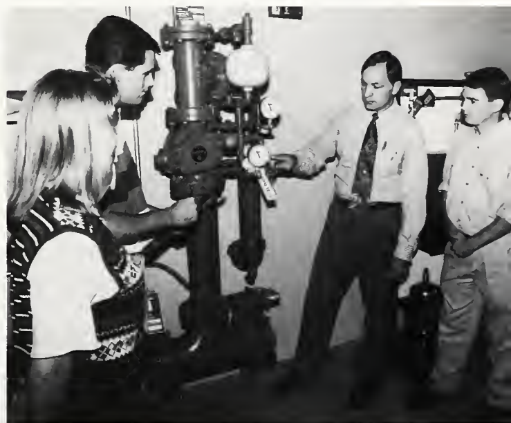
Instructor, Larry Collins demonstrates the sprinkler system to students.
