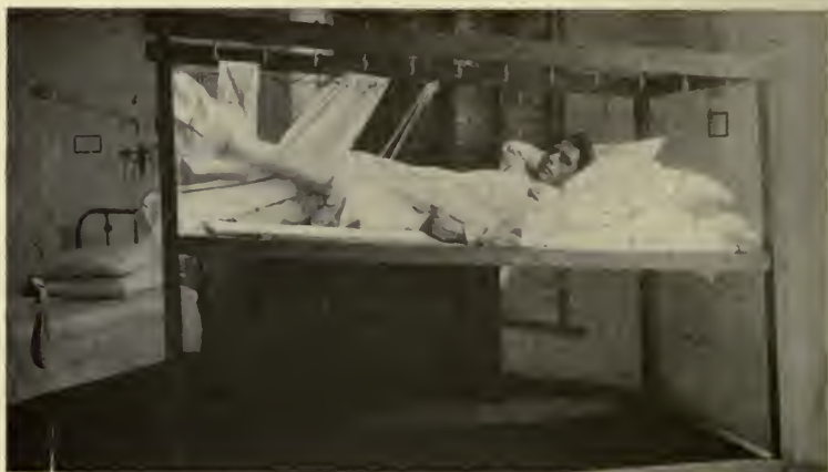
FIG. 94. Shows suspension frame for fracture of the thigh. This frame was constructed in order to facilitate dressings, as the thigh was very badly infected and any movement caused extreme pain to the patient. A Bradford frame is supported on two crossbars and over the frame is a hammock which can be suspended to the hooks on the upper bar. When it is required to do a dressing the hammock is caught over the hooks, the Bradford frame is dropped out and the patient remains suspended. By this method the wound is freely accessible for dressing, while at the same time the patient is disturbed very little.
