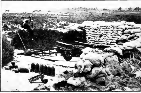
RAMPARTS THAT BAFFLED McCLELLAN. (Hasty fortifications of the Confederates at Yorktown.) It was against such fortifications as these, which Magruder had hastily reinforced with sand-bags, that McClellan spent a month preparing his heavy batteries. Magruder had far too few soldiers to man his long line of defenses properly, and his position could have been taken by a single determined attack. This rampart was occupied by the Confederate general, D. H. Hill, who had been the first to enter Yorktown in order to prepare it for siege. He was the last to leave it on the night of May 3, 1862.
