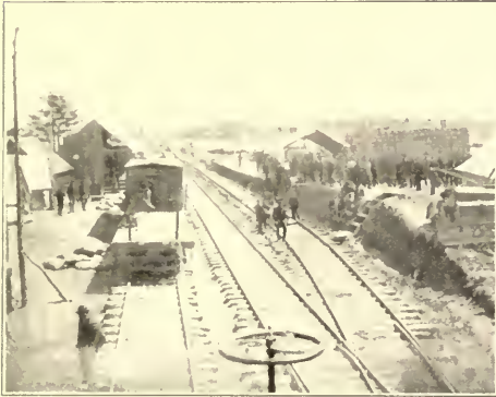
STORES AT STONEMAN'S STATION
