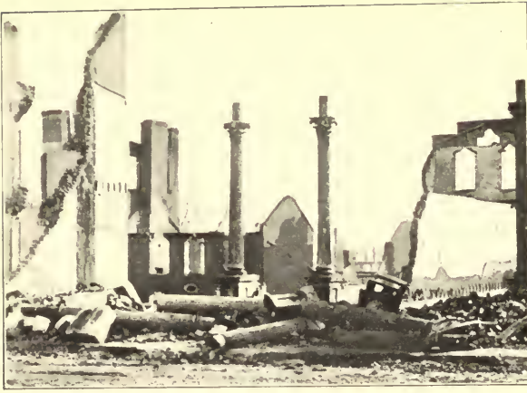
SOUTHERN EXPRESS OFFICE, RICHMOND
