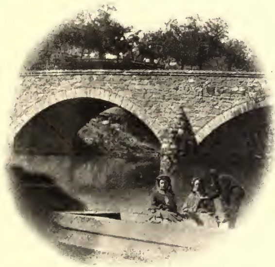
AT ANTIETAM BRIDGE
