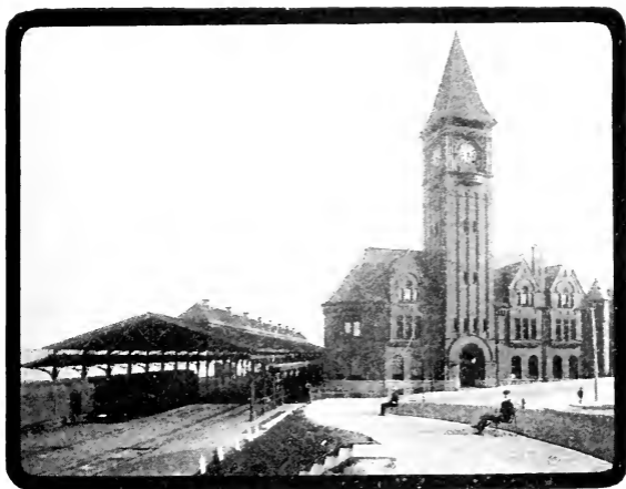
CHICAGO & NORTHWESTERN RY. STATION. FACING LAKE AND JUNEAU PARK.
