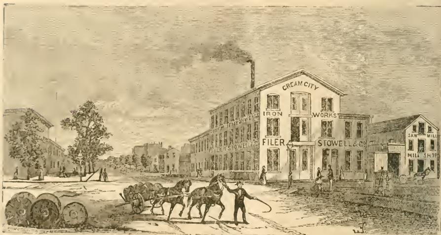
CREAM CITY IRON WORKS.
