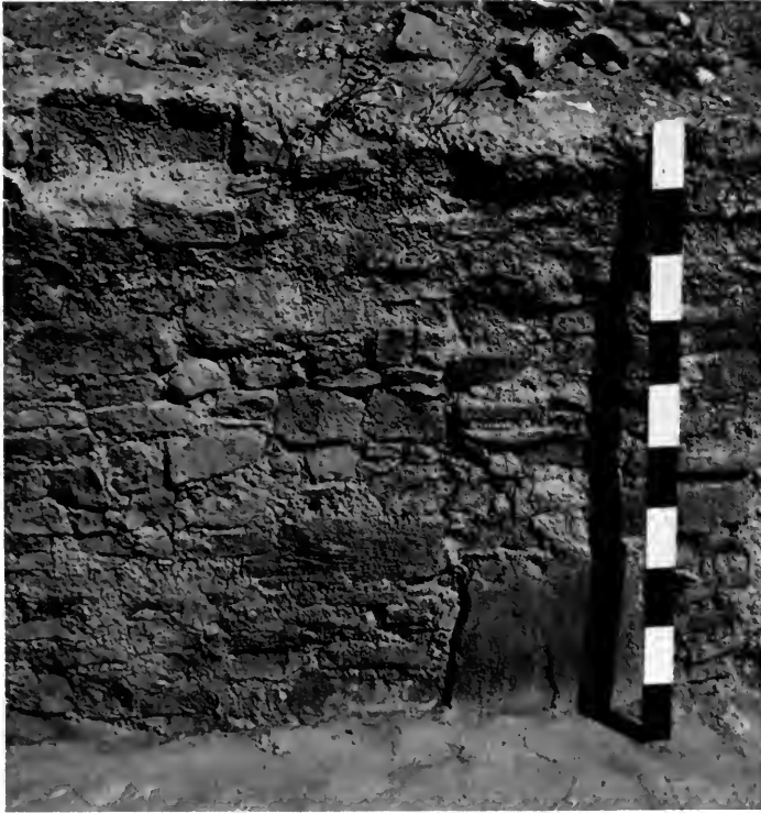
FIG. 15. Rubble masonry (Type II) in north wall of Room 13A, Hooper Ranch Pueblo. Meter stick at right.
