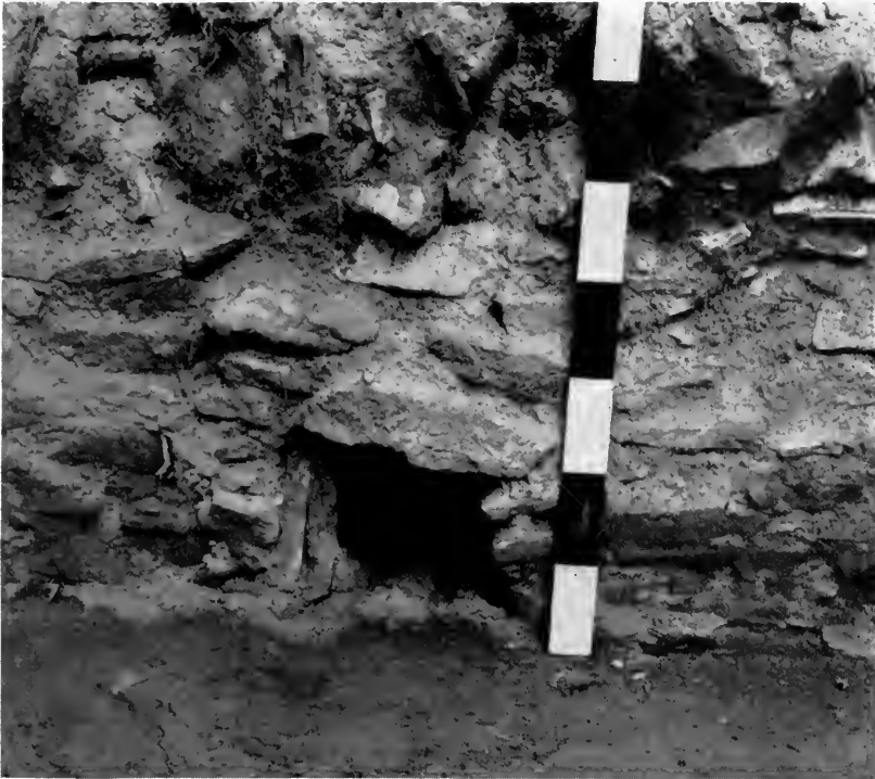
FIG. 18. Ventilator through partition wall between Rooms 8A and 12A, Hooper Ranch Pueblo, showing construction of lintel and sides. Meter stick at right.
