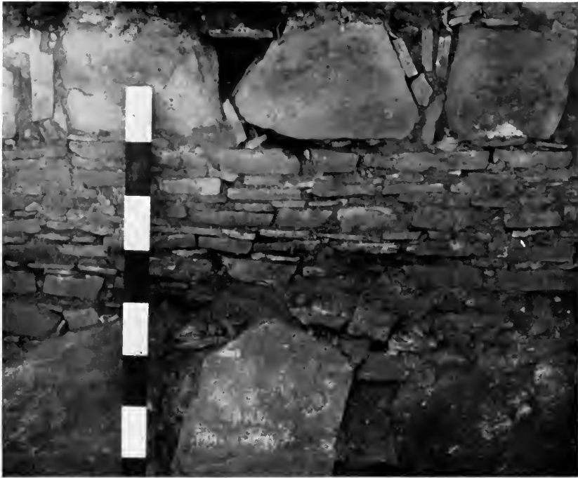
FIG. 27. Masonry of Type I (slabs set on edge) in east wall of Kiva I, Hooper Ranch Pueblo. Meter stick at left.
