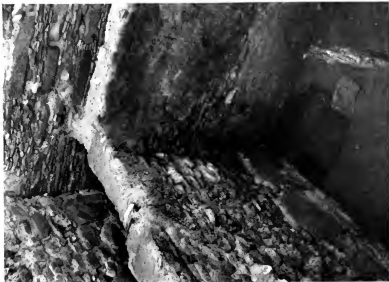
FIG. 31. Diagonal bond, northwest corner of Room 2B, Hooper Ranch Pueblo. Height of wall above pit, 155 cm.
