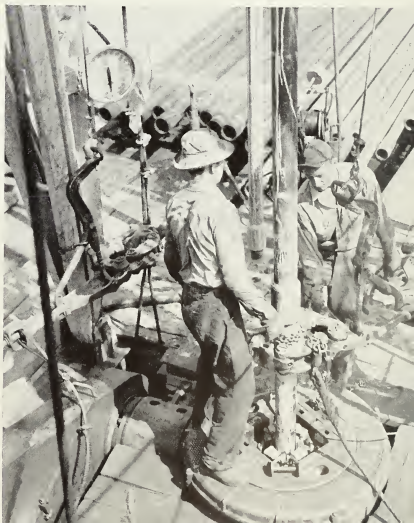
Scene on rig floor of rotary-drilled oil well
