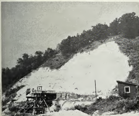
Pit producing chert gravel for road material—Alexander County, Illinois.
