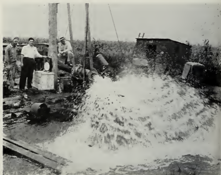
Water well in Champaign-Urbana area located by the Illinois Geological Survey through the earth resistivity method. (Champaign-Urbana Courier photo.)
