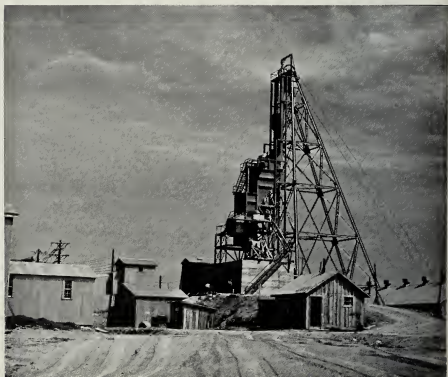
Head frame for bringing zinc ore to the surface at a northwestern Illinois mine and plant for separating ore from waste rock.
