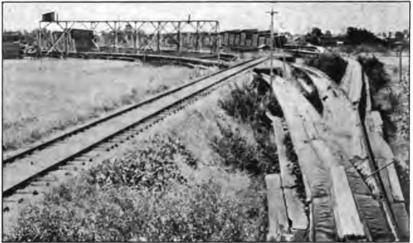
Photo No. 24. "V" Flume for transporting lumber, Madera Sugar Pine Company, Madera County, California.
