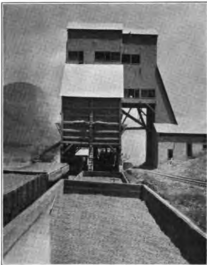
Photo No. 32. Loading railroad cars at Kings River Quarry, Piedra, Fresno County.
