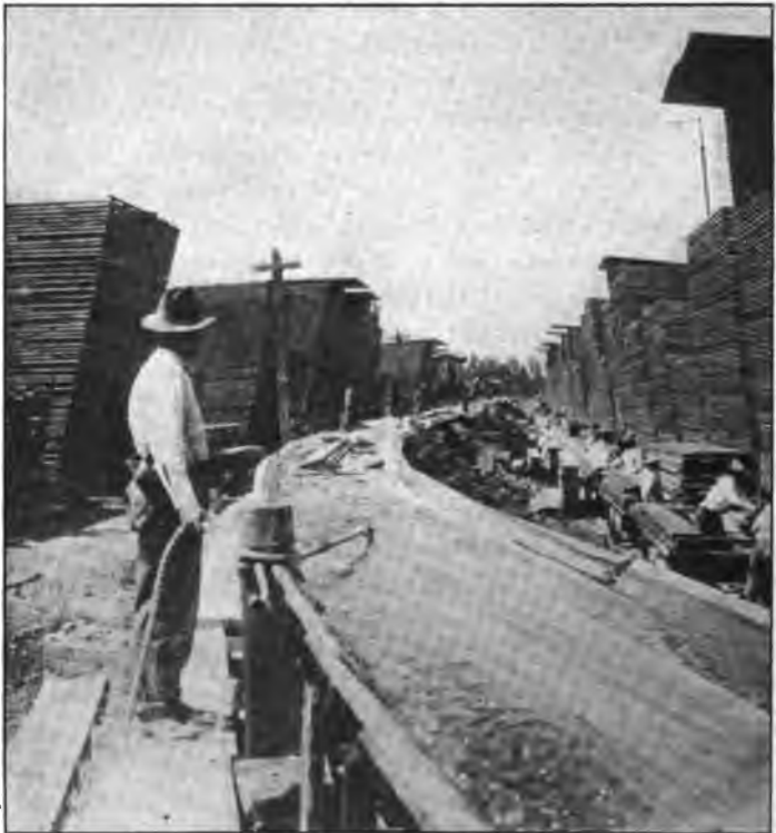
Photo No. 22. Discharging lumber from "V" flume, Madera Sugar Pine Company, Madera County, California.
