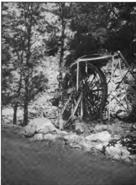
Photo No. 8. Water wheel operating "Marathon" tube mill, Golden Group.
