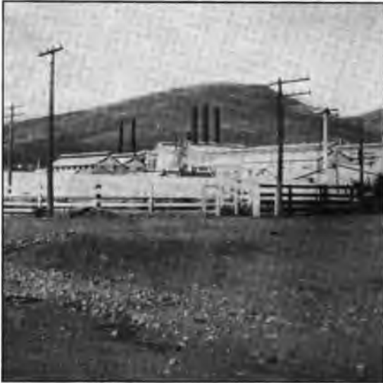
Photo No. 4. Cement plant at Monolith, erected by City of Los Angeles.
