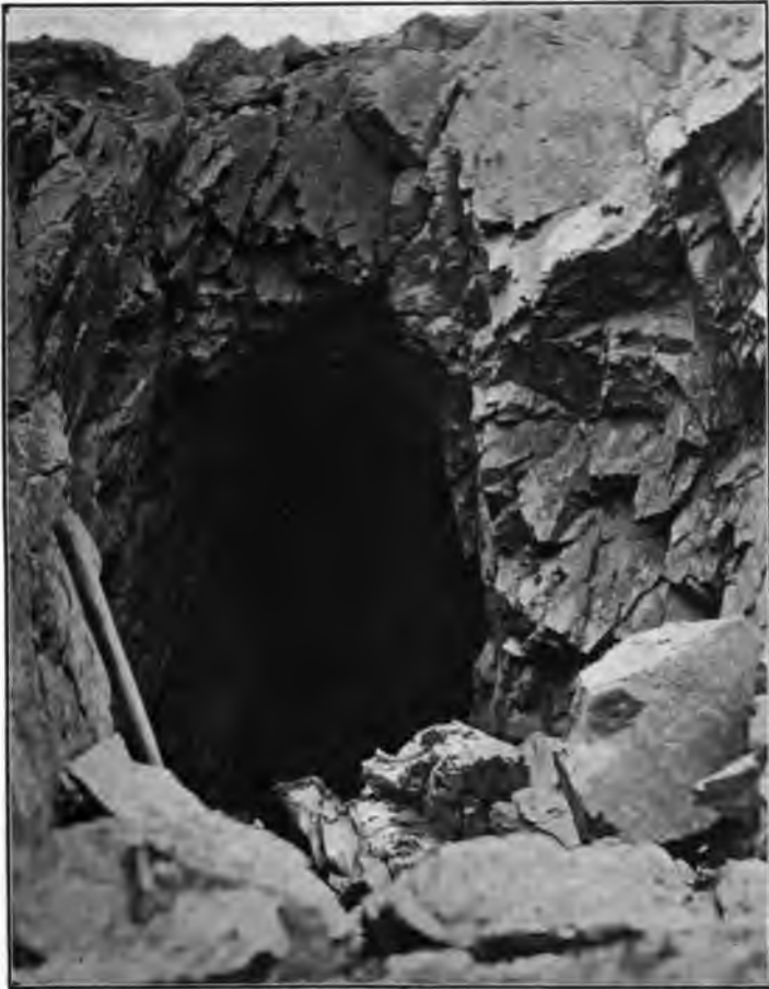
Fig. B. Portal of tunnel in massive iron ore on Iron Mountain. Photo by F. B. Weeks.
