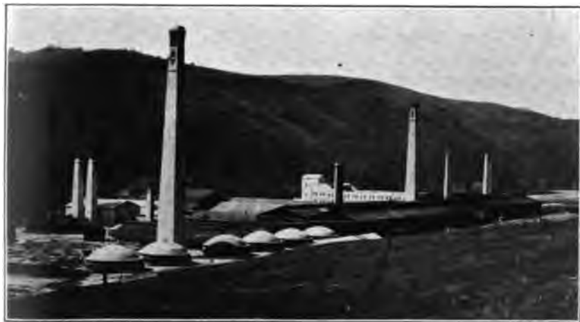
Carnegie Brick and Pottery Company's Plant at Carnegie, San Joaquin County, California. Photo by Walter W. Bradley.
