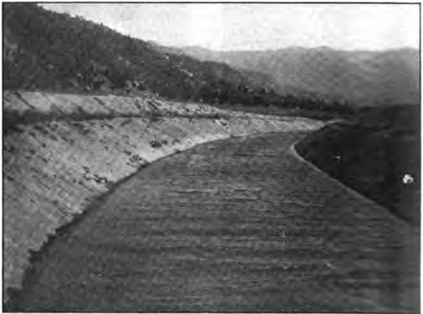
Photo No. 3. Canal, Pacific Light and Power Company.
