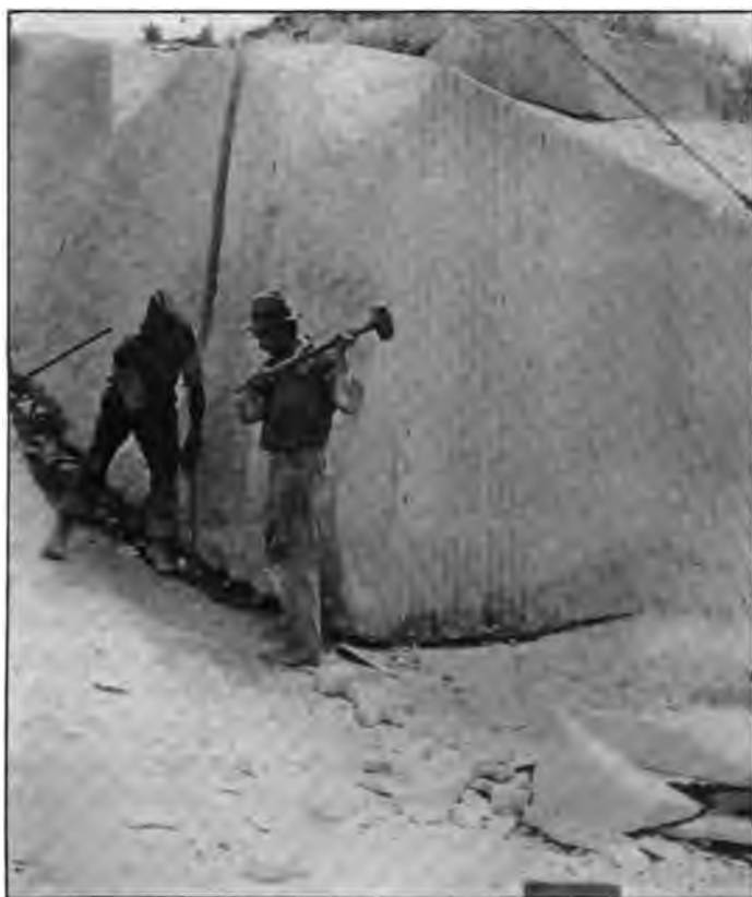
Photo No. 2. Wedging out a large block of granite (about 10 feet by 20 feet by 5 feet). Raymond Granite Company, Madera County, California.
