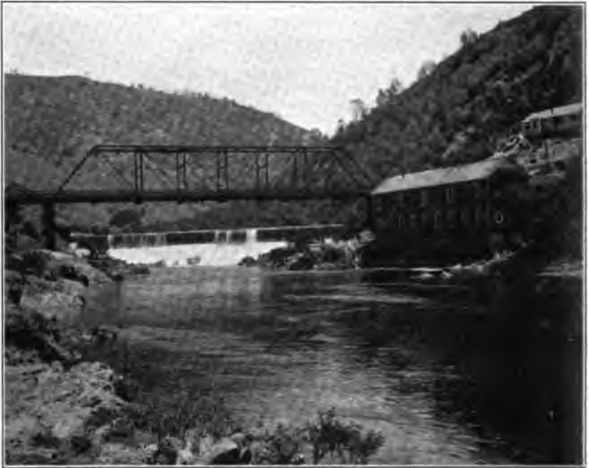
Mariposa Commercial and Mining Company's dam and hydroelectric plant on the Merced River at Bagby, Mariposa County, California.
