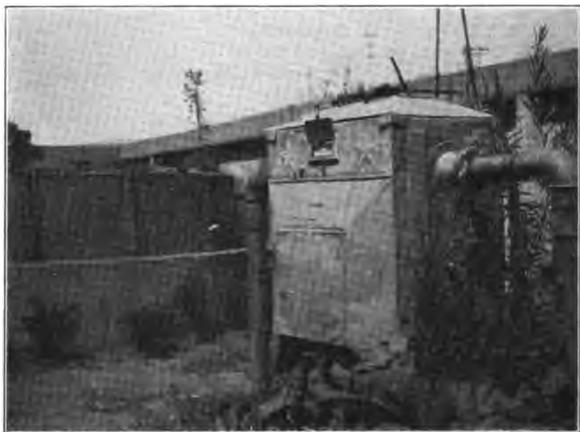
Gasometer and meter of a natural gas well in Stockton, belonging to the Western States Gas and Electric Company.
