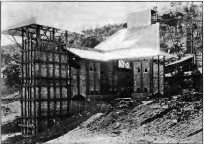
Photo No. 116. Ten-ton Scott fine-ore furnace and condensers, Kings Quicksilver Mining Company, Ltd., Kings County, California.
