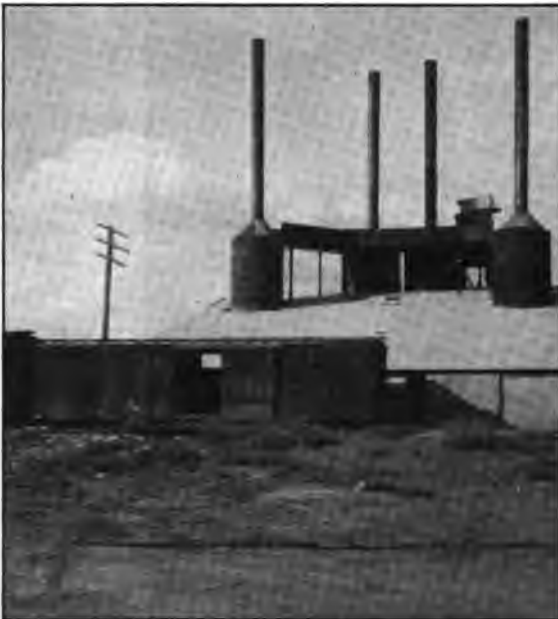
Photo No. 12. Summit Lime Company's Plant at Tehachapi.
