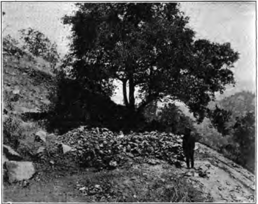
Copper dump on the property of the Indian Peak copper claims, Mariposa County, California.
