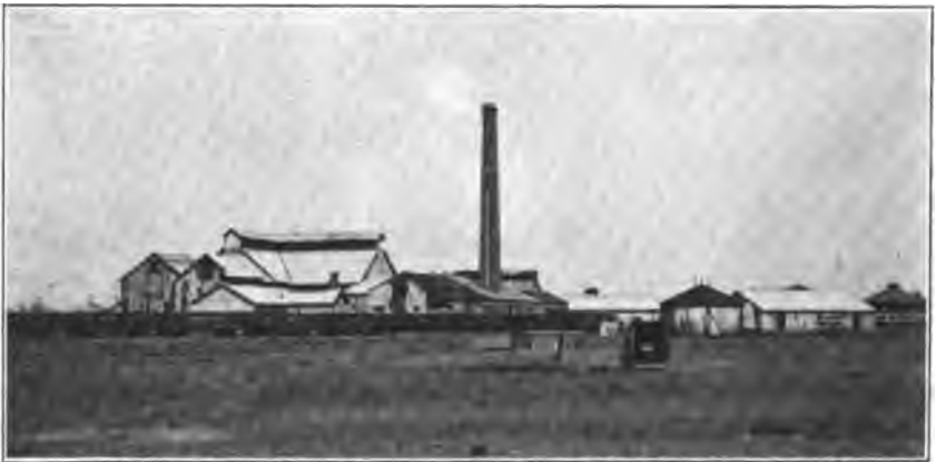
Stockton Window Glass Plant at Stockton, San Joaquin County, California, owned by the Western States Gas and Electric Company.
