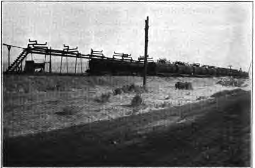
Photo No. 114. Oil loading rack, Crump Siding near Coalinga, Fresno County.
