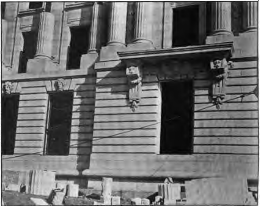
Photo No. 129. Sculptural detail on City Hall, San Francisco. Stone from McGilvray Raymond Granite Company, Madera County, California.
