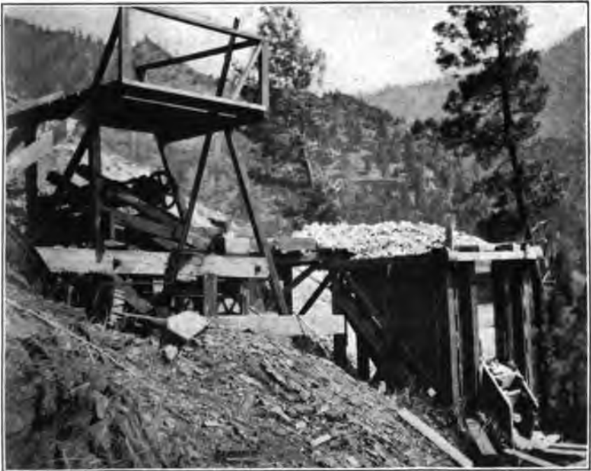
El Portal Mining Company's barytes quarry on the Merced River one mile below El Portal, Mariposa County, California.
