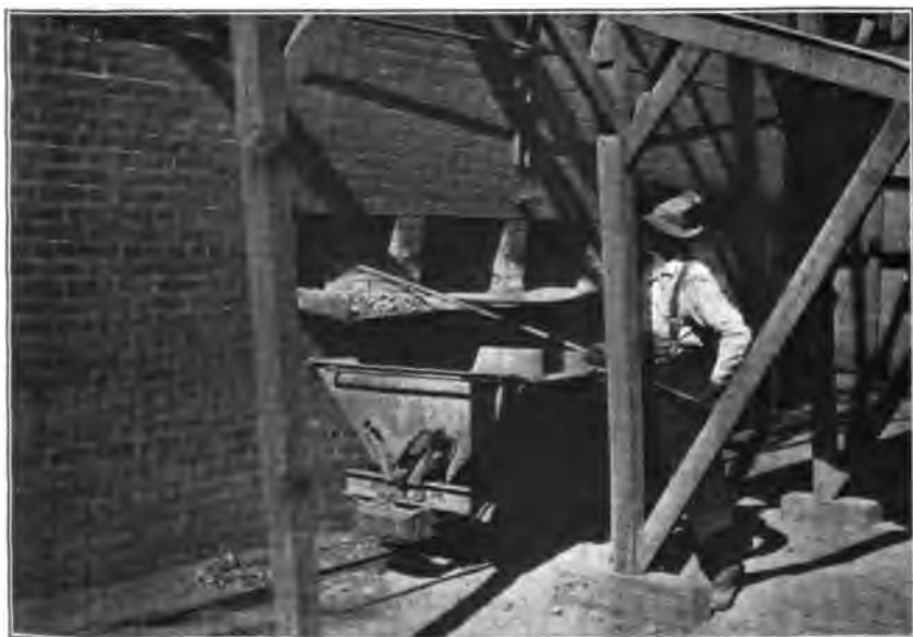
Photo No. 107. Drawing off burned ore, Pacific Quicksilver Mine, Fresno County.
