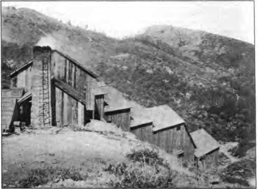
Photo No. 19. Fifty-ton Scott furnace at the Helen Mine, near Middletown, Lake County, California. Old dumps of the Wall Street Mine in the distance.
