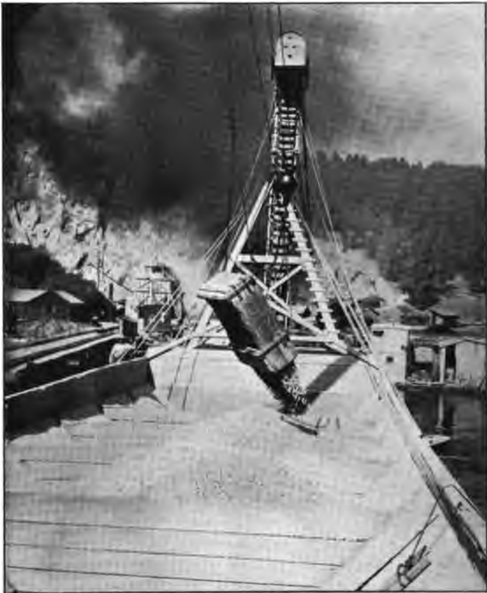
Photo No. 120. Barge "San Pablo" (self-dumping) of San Francisco Quarries Company at pier, Marin County, California. Showing bin arrangement.
