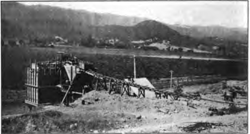
Photo No. 33. Crusher and bins at Napa County Rock Plant, near Yountville.
