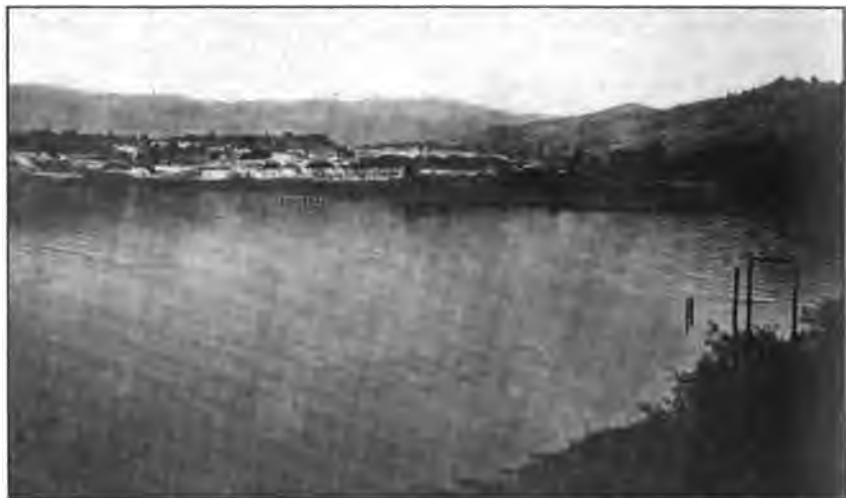
Photo No. 22. Sulphur Bank Mine from lake side.
