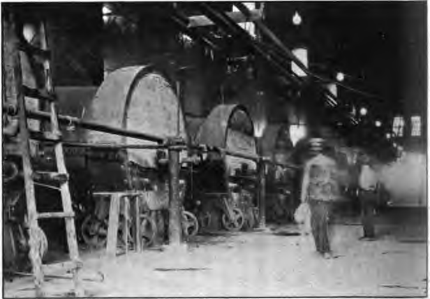
Photo No. 69. Rotary kilns in new mill of Pacific Portland Cement Company, Solano County.
