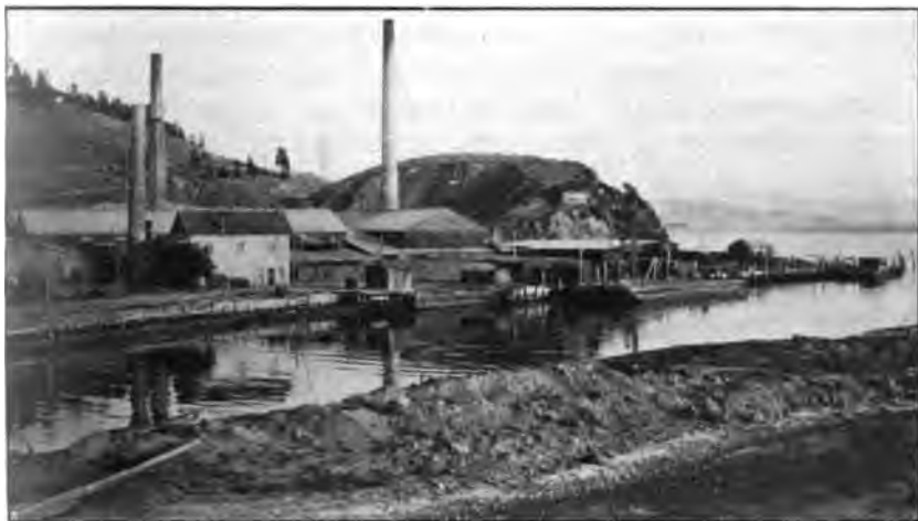
Photo No. 131. Plant and furnaces of the McNear Brick Company, near San Rafael, Marin County, California.
