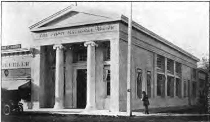
Photo No. 153. First National Bank Building, Healdsburg, California. A concrete building finished with a magnesite paint.
