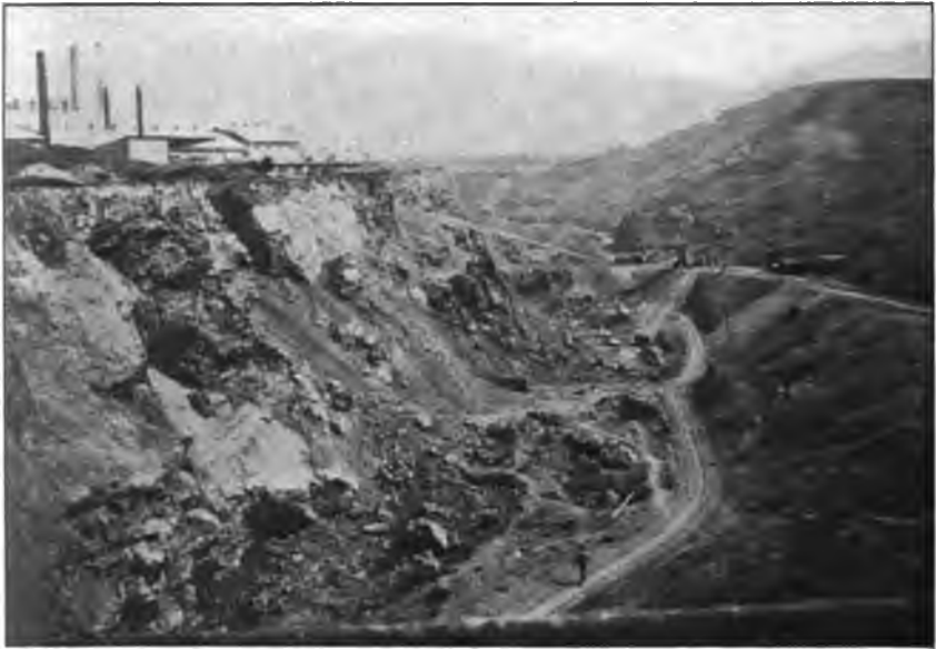
Photo No. 44. Clay pit of the Standard Portland Cement Company, Napa Junction, Napa County.
