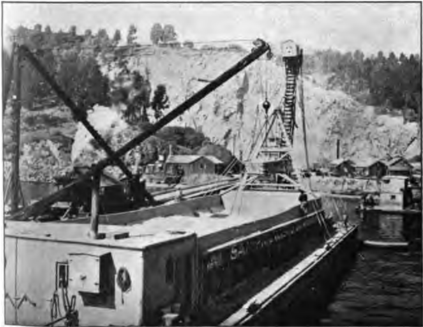
Photo No. 121. Barge "San Pablo" of San Francisco Quarries Company, at pier. Side view.
