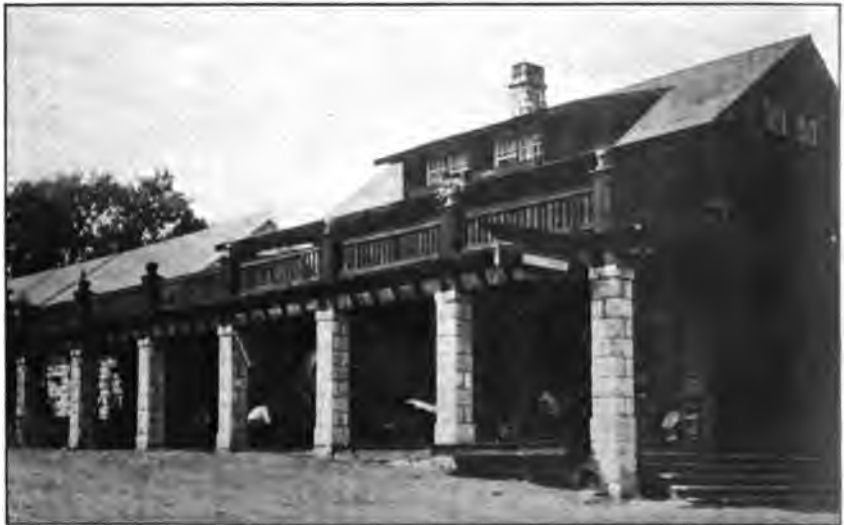
Photo No. 17. Hotel at Seigler Hot Springs, Lake County, California.
