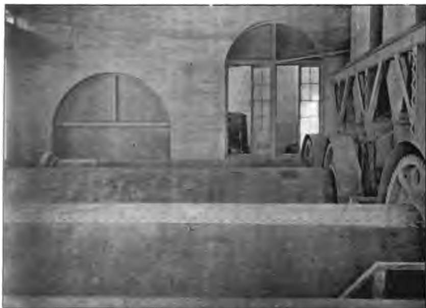
Photo No. 51. Final tube mills in mill of Standard Portland Cement Company, Napa Junction, Napa County.
