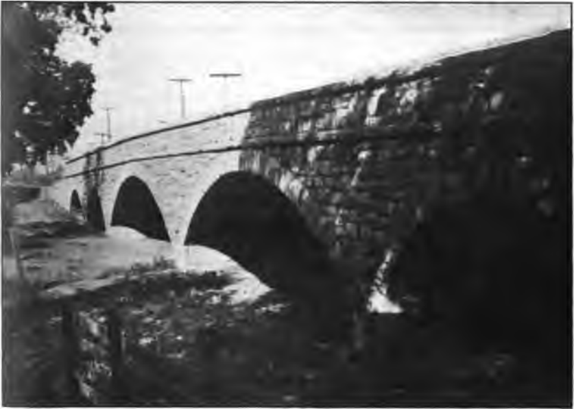
Photo No. 35. "Little Trancas" bridge, near Napa, Napa County. Stone from Wing Quarry, 1908.
