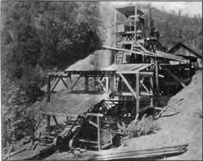
Photo No. 29. Mill at Aetna Quicksilver Mine, Napa County.
