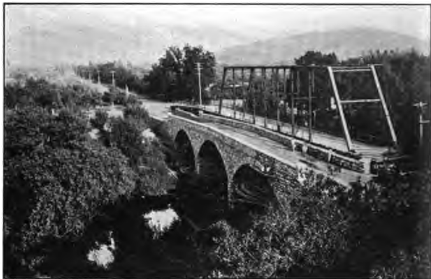
Photo No. 43. "Big Trancas" bridge near Napa, Napa County. Stone from Wing Quarry, 1913.
