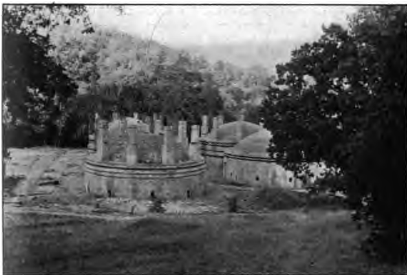
Photo No. 135. Circular Brick Kilns of California Brick and Pottery Company, Glen Ellen, Sonoma County.
