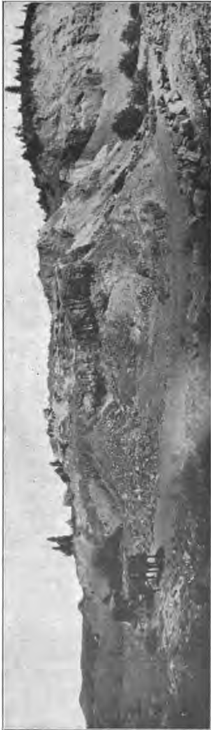
Photo No. 7. Old hydraulic workings of the Port Wine channel, showing basalt sheets in gravel bank.
