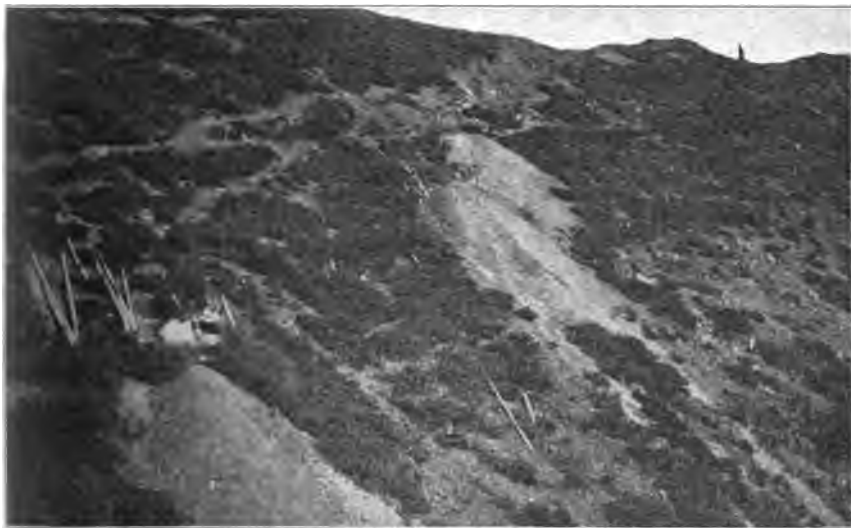
Photo No. 19. Open cut along outcrop of Sierra Buttes lode.
