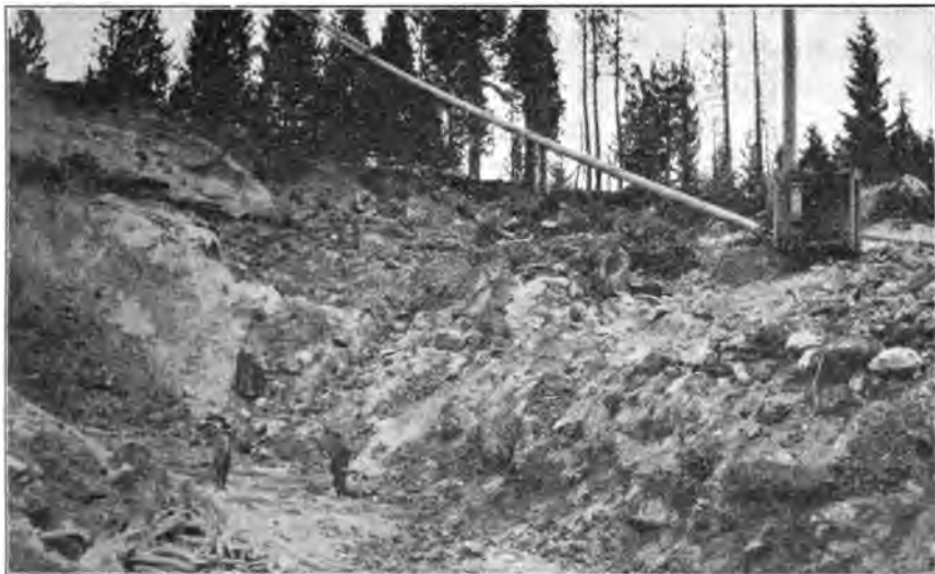
Photo No. 10. Lava-capped channel at Scales. Shows derrick used for handling large boulders.
