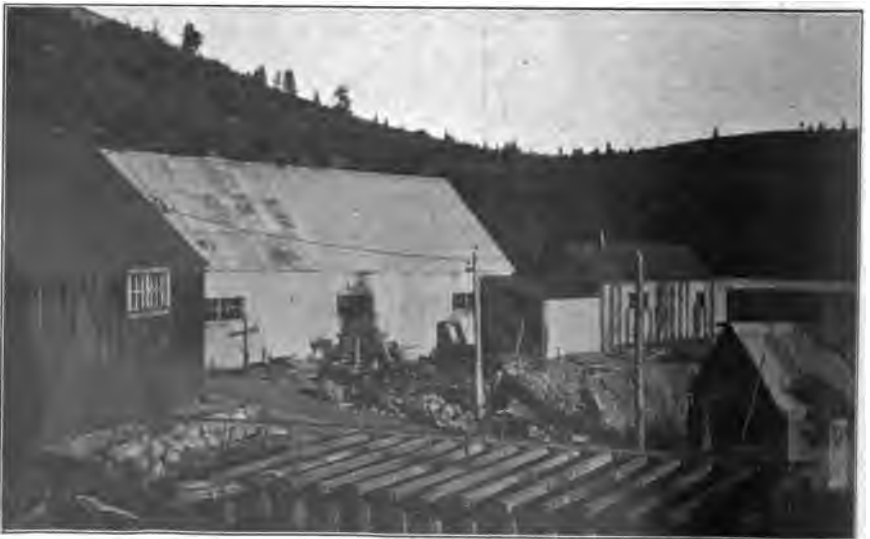
Photo No. 17. Surface plant at North Fork mine.
