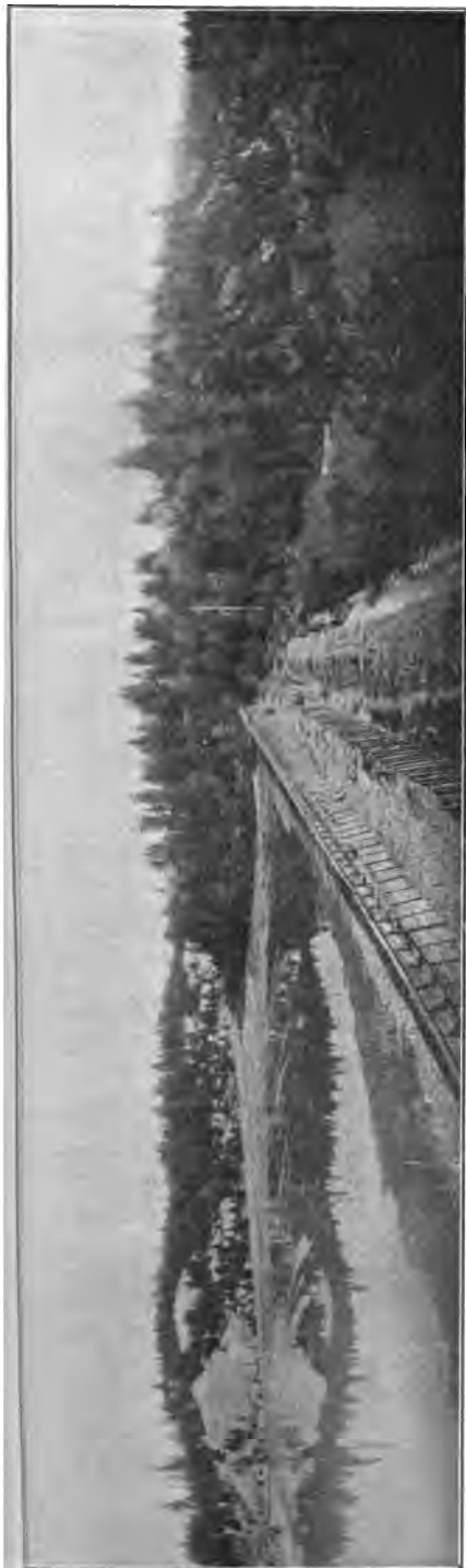
Photo No. 14. Brandy City hydraulic mine. Shows tailing impounding dam built of hydraulic debris.
