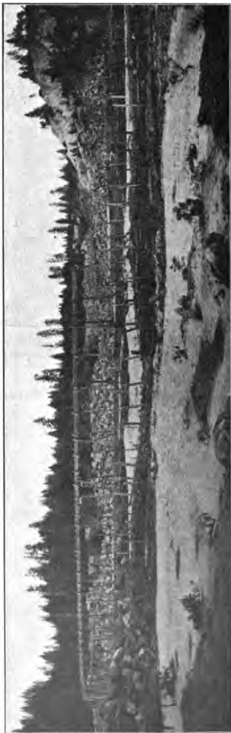
Photo No. 14. Brandy City hydraulic mine. Shows tailing impounding dam built of hydraulic debris.
