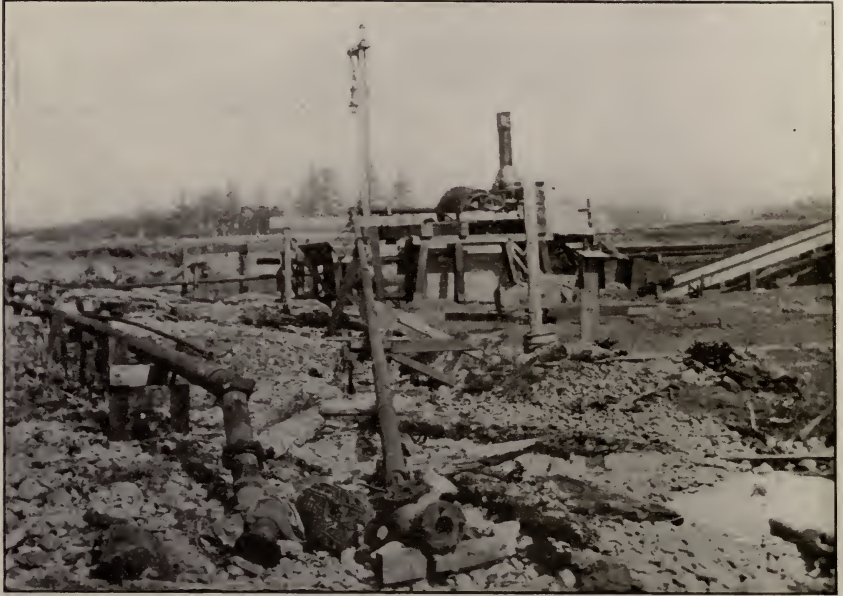
Oro Del Norte Black Sands Plant, showing suction pipe line.
