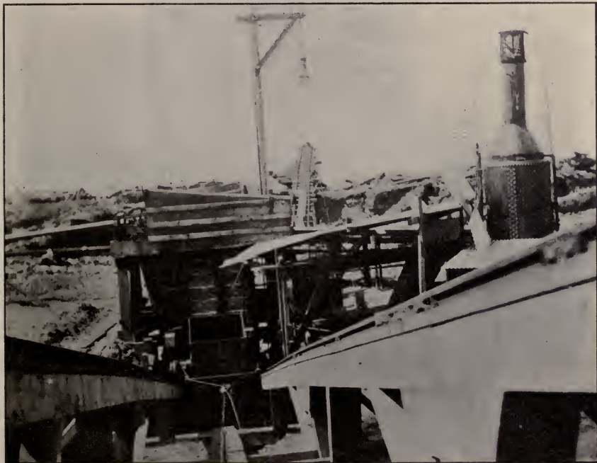
Oro Del Norte Black Sands Plant, showing sand skip and track for dumping waste.
