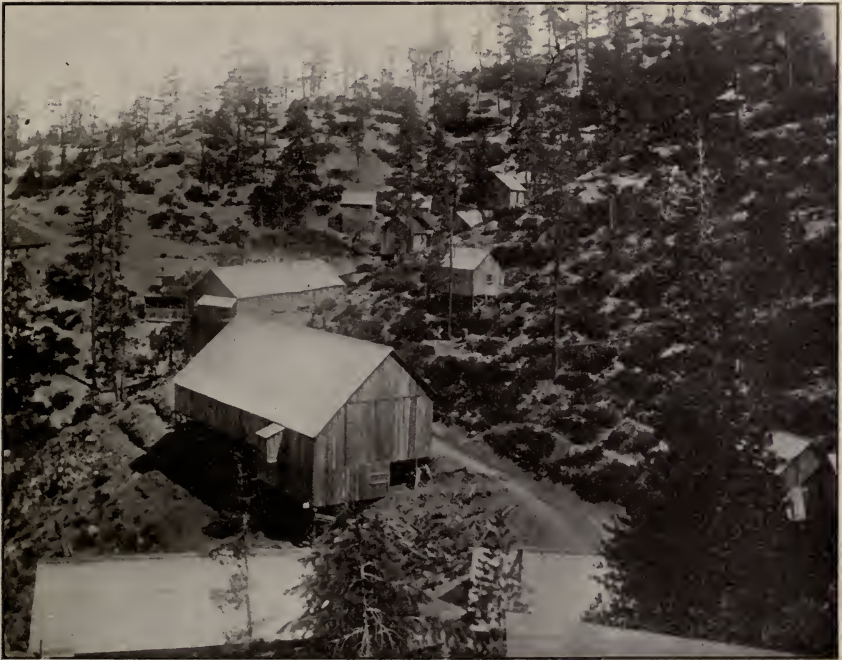
Camp buildings of the Horse Mountain Copper Mining Company, on Horse Mountain, Humboldt County, California.
