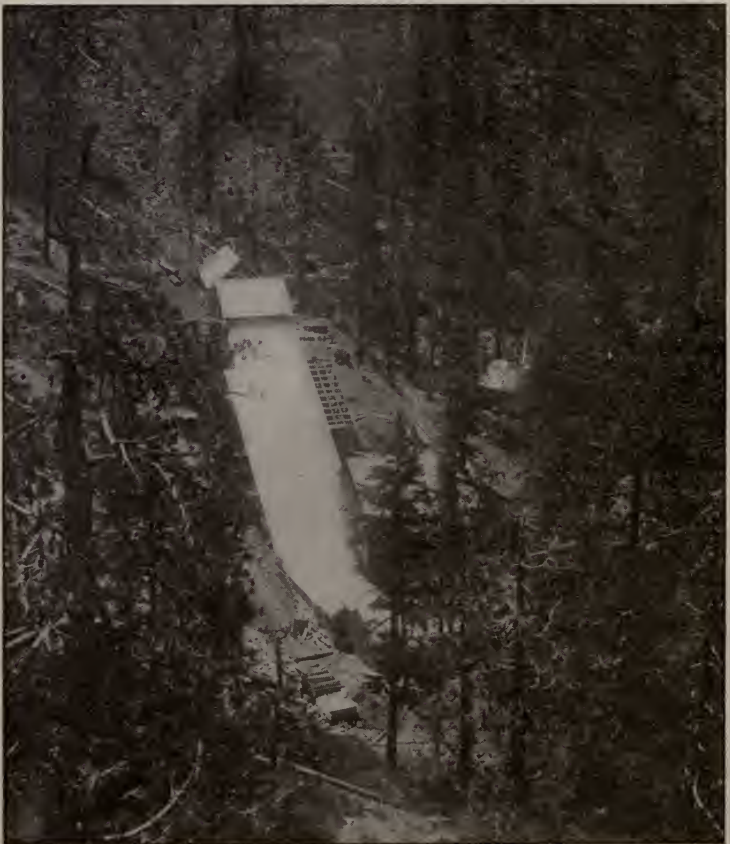
Mill of the Horse Mountain Copper Mine, Humboldt County, California.
