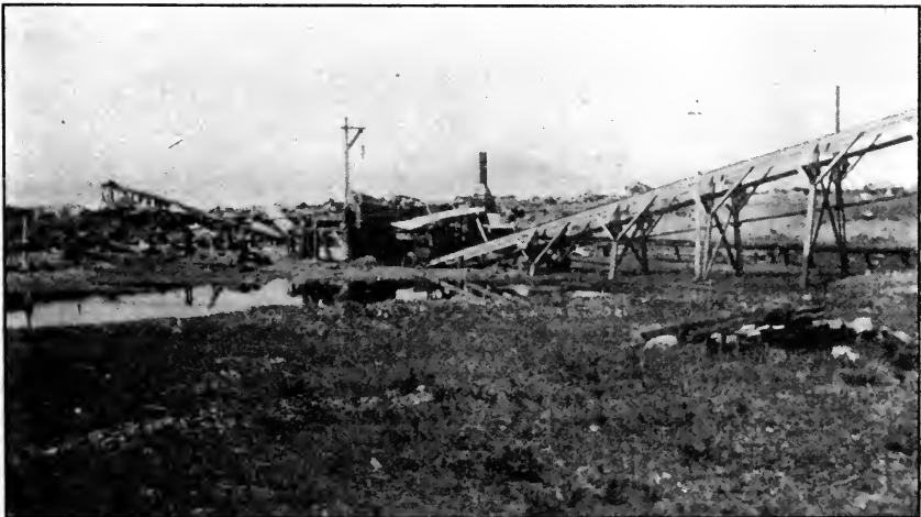
Oro Del Norte Black Sands Plant, showing method of hauling sands to bins on incline trestle. 2—B14456
