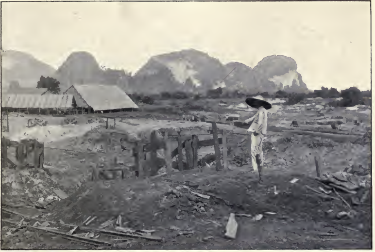
SUBSIDED WORKINGS, TAMBUN MINE, PERAK.
