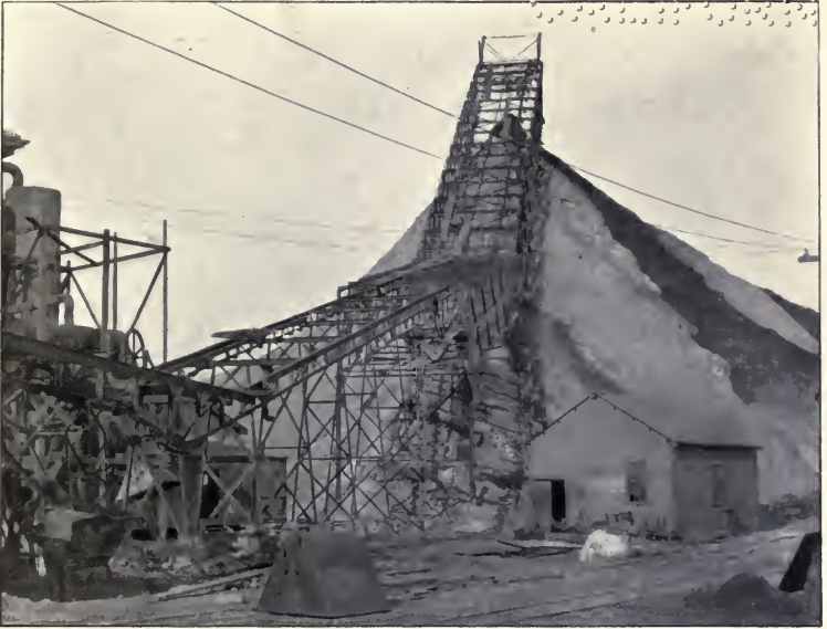
GREAT BOULDER TAILINGS ELEVATOR.
