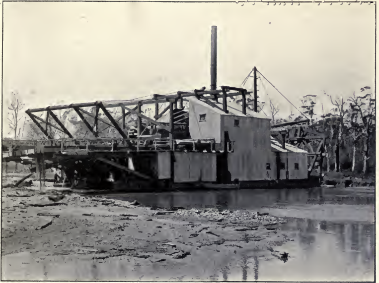
RINGAROOMA BUCKET DREDGE.
