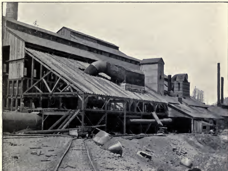
LARGE SMELTING FURNACE, DOMINION COMPANY.
