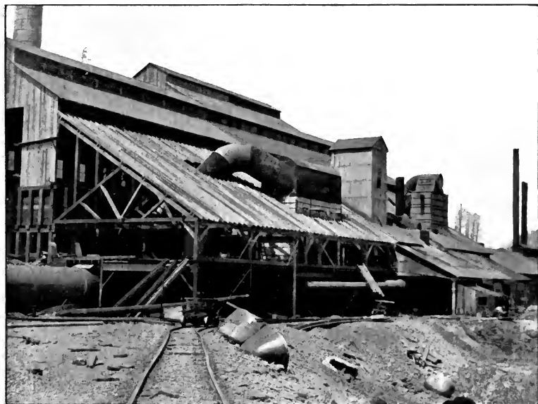
LARGE SMELTING FURNACE, DOMINION COMPANY.
