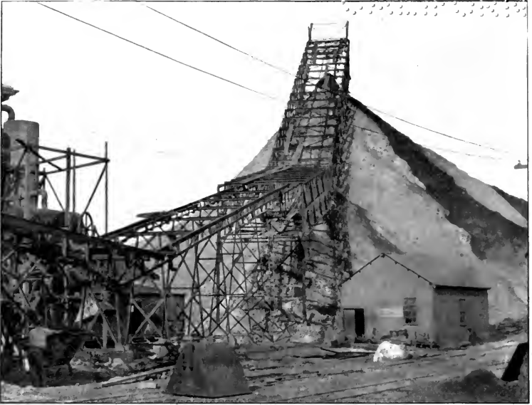
GREAT BOULDER TAILINGS ELEVATOR.
