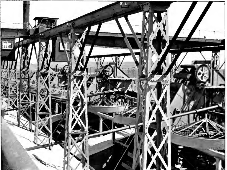
PREMIER NO. 3 WASHING PLANT.
