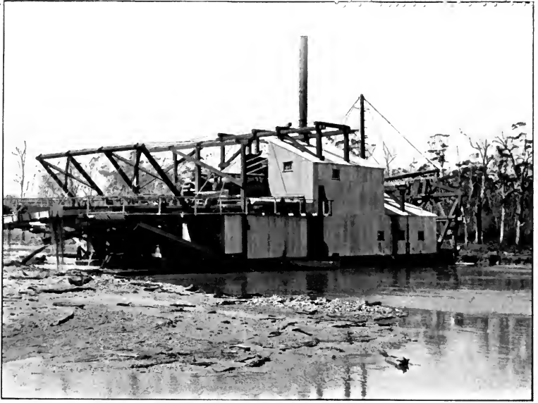
RINGAROOMA BUCKET DREDGE.
