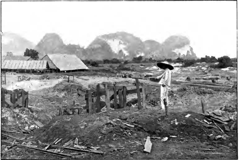
SUBSIDED WORKINGS, TAMBUN MINE, PERAK.
