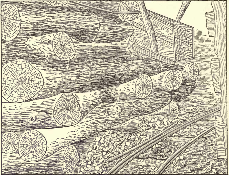
FIG. 97. — A TYPICAL MILL CHUTE.
