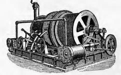
1, 2 or 4 Drums, with Reversible Link Motion or Patent Improved Friction. Made only by the
