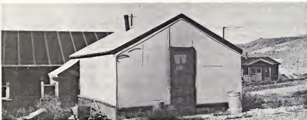
P.R. Bradley's house at Opalite, Nevada in 1931 - note double roof, canvas walls - Boarding house in the background - at right.
