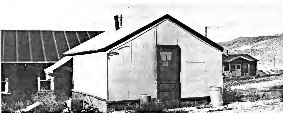
P.R. Bradley's house at Opalite, Nevada in 1931 - note double roof, canvas walls - Boarding house in the background - at right.
