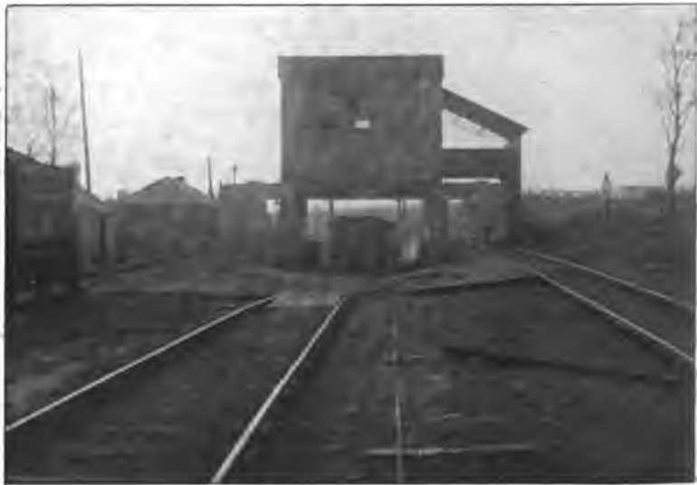
FIG. 14.—EASTERN FRONT OF DRUM-HOUSE.
