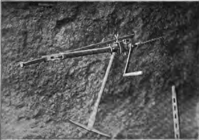
FIG. 11.—GRAY-TABBIT ROTARY DRILLING-MACHINE.
