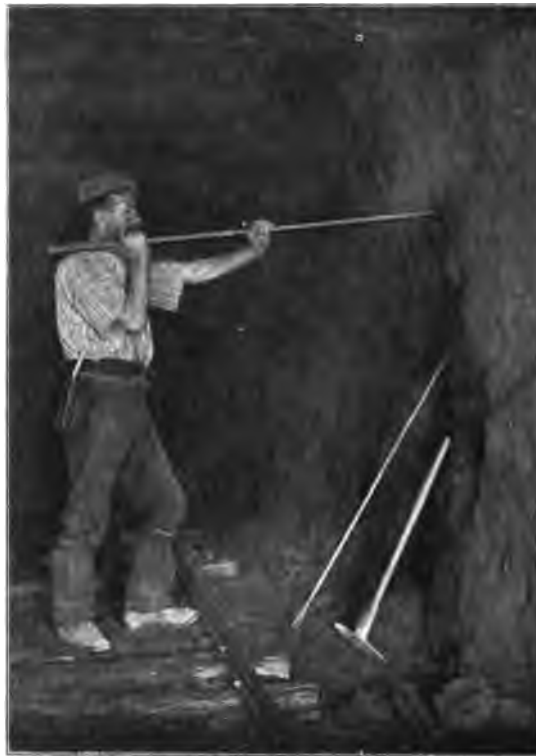
FIG. 16.—MINER USING A JUMPER-DRILL.
