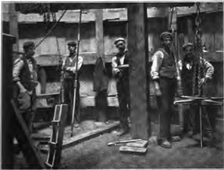
FIG. 6.—BORING HOLES FOR FREEZING-PIPES.
