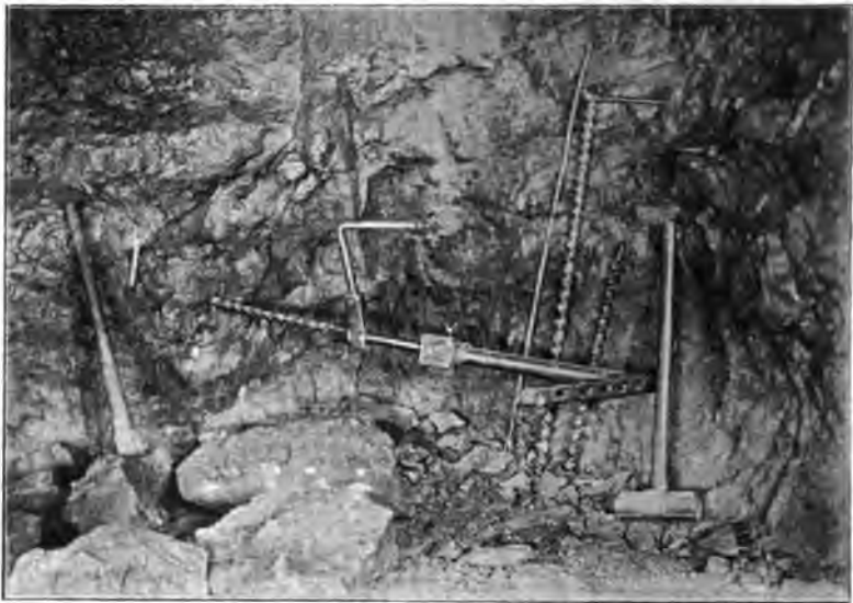
FIG. 8.—HARDY RATCHET DRILLING-MACHINE.
