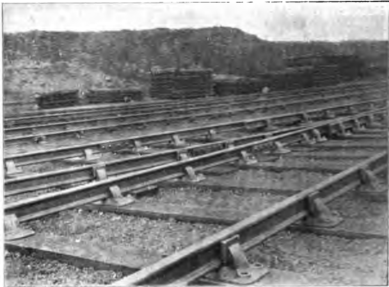
FIG. 2. —THE IMPROVED IRON WEDGE APPLIED TO CROSSINGS.
