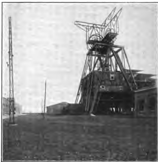
FIG. 12.—DOUBLE HEADGEAR AT RHEIN-ELBE COLLIERY.
