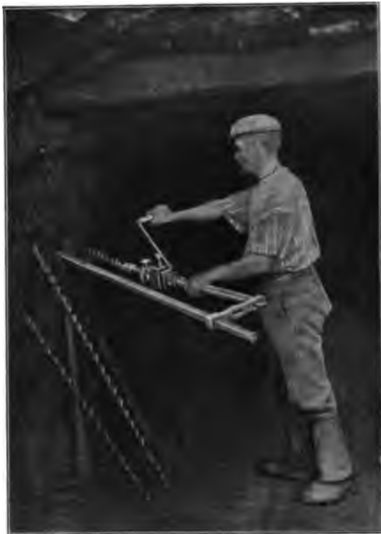
FIG. 10.—GRAY-TARBIT ROTARY DRILLING-MACHINE.
