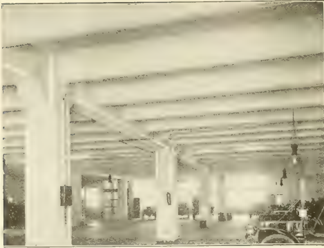
2. KAHN SYSTEM SOLID CONCRETE SLABS AND BEAMS.
