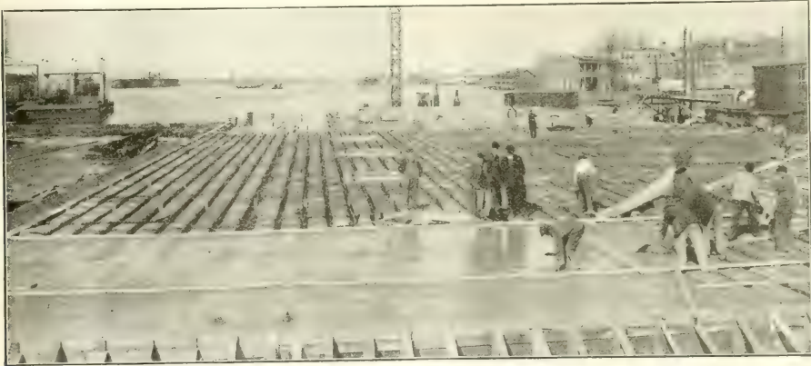
1. STEEL FLOOR IN CONSTRUCTION.
