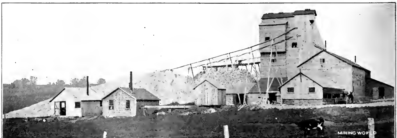
PLANT AT THE BULL MOOSE MINE, WISCONSIN.
