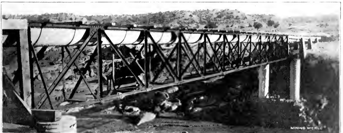
METAL WATER FLUME IN NEW MEXICO FOR U. S. INDIAN SERVICE.
