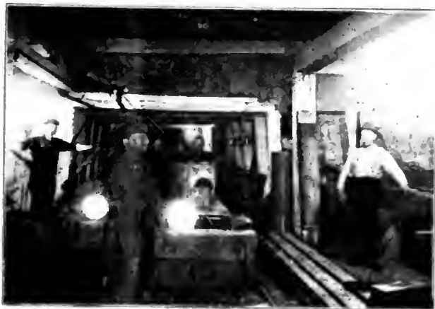
TWO ELECTRIC 3-TON MOTORS IN FOREGROUND, SILVER HILL STATION.
