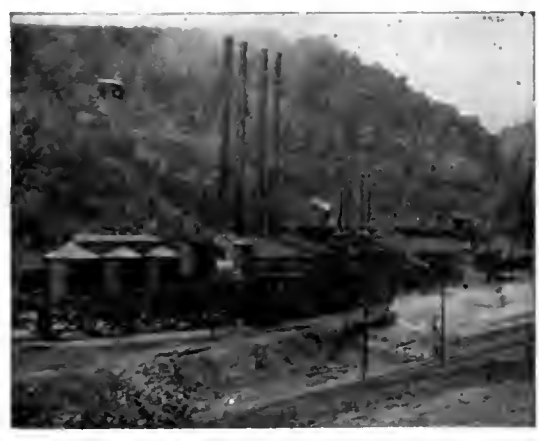
SOFTENER INSTALLATION, U. S. COAL & OIL CO., HOLDEN, W. VA. (BOILER FEED AND MUNICIPAL).
