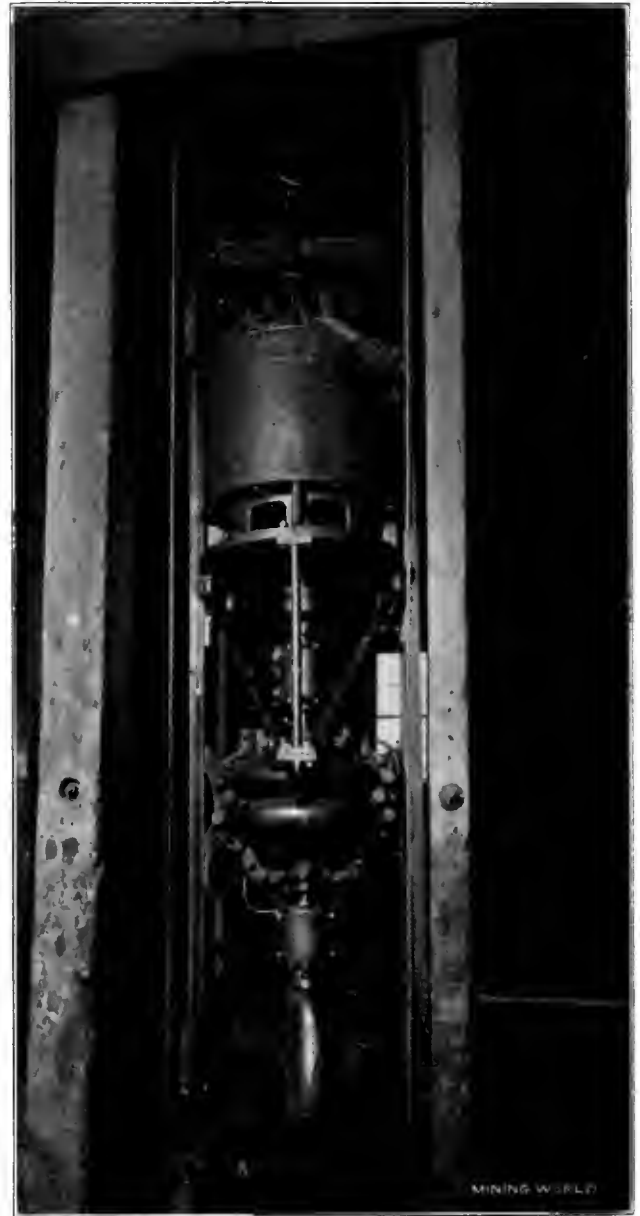
PROVIDENCE 2-STAGE SINKING PUMP.
