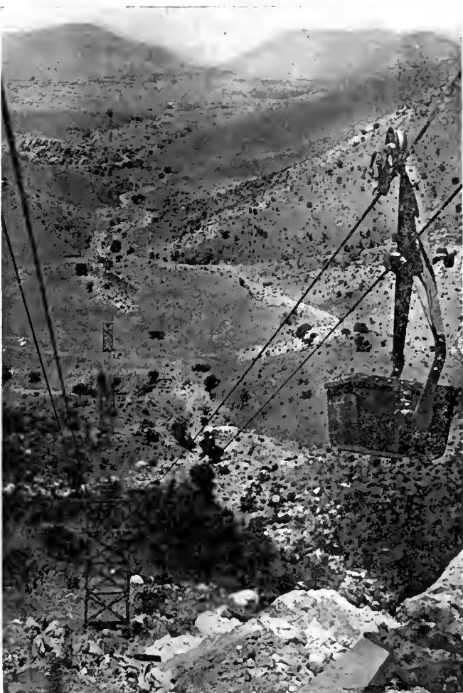
TRAM LEADING FROM MINE TO RAILROAD.
