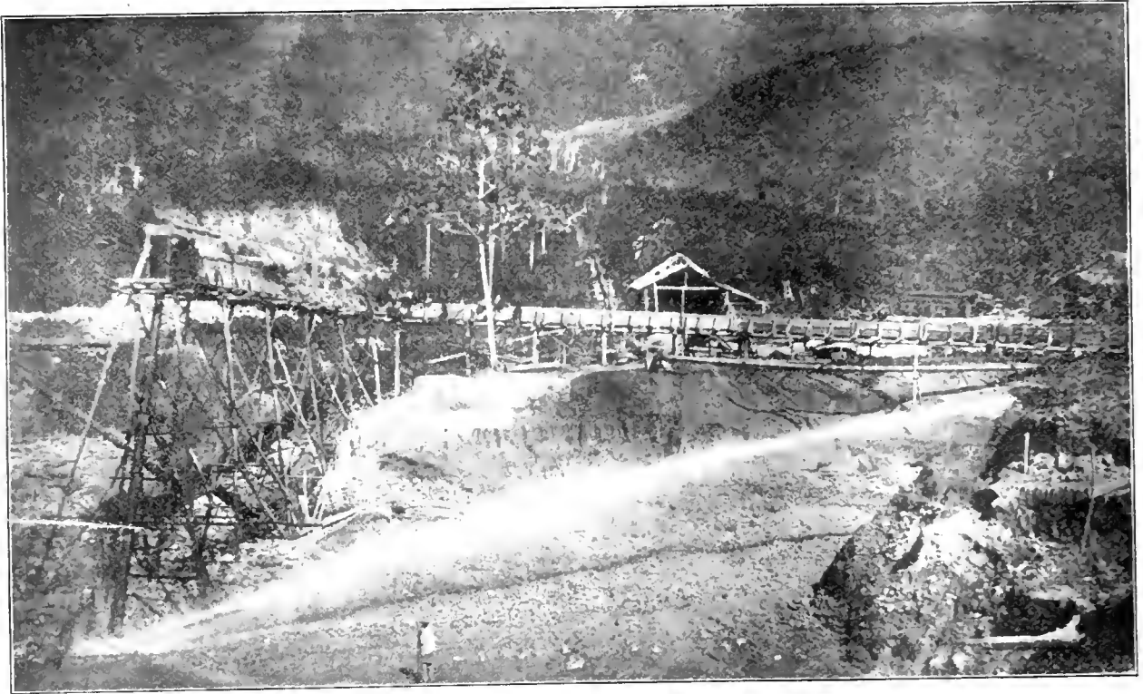
MONITOR IN OPERATION AT HYDRAULIC ELEVATOR IN COLOMBIA ON RIO GRANDE.
