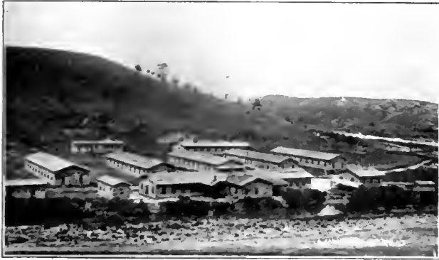
MINERS' HOUSES OF TENNESSEE COPPER CO.
