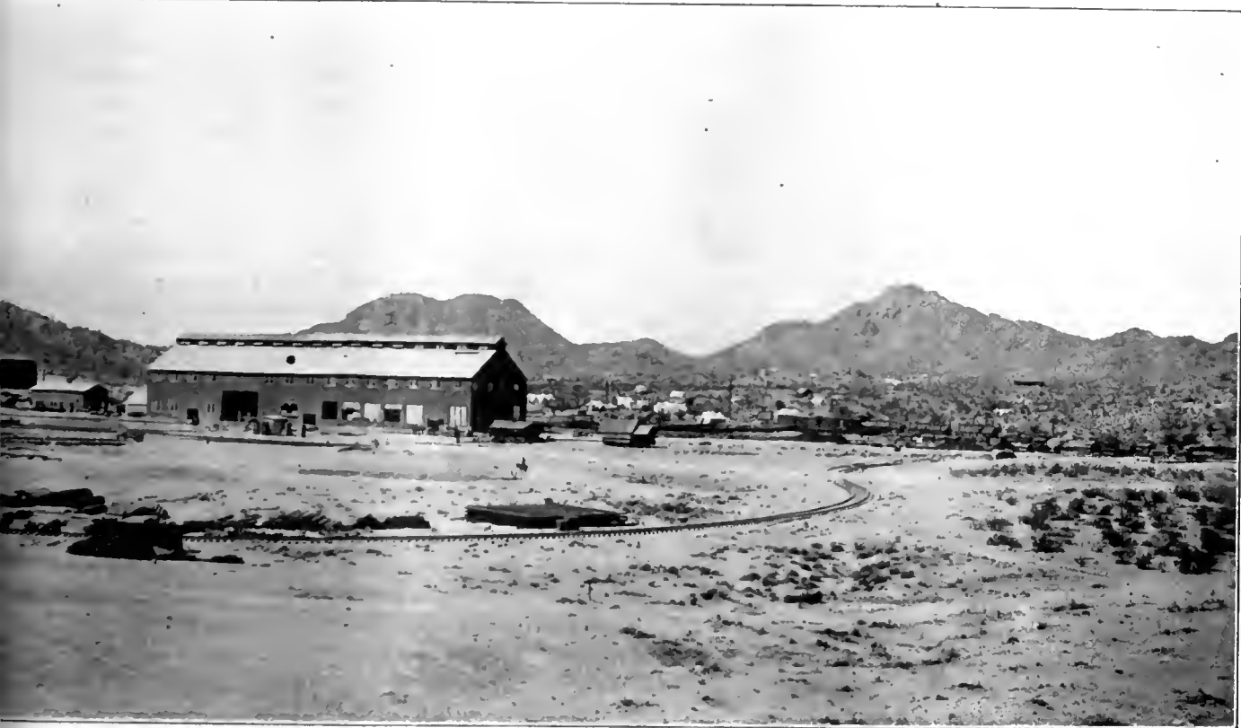
Oil Tanks. Machine Shop.
