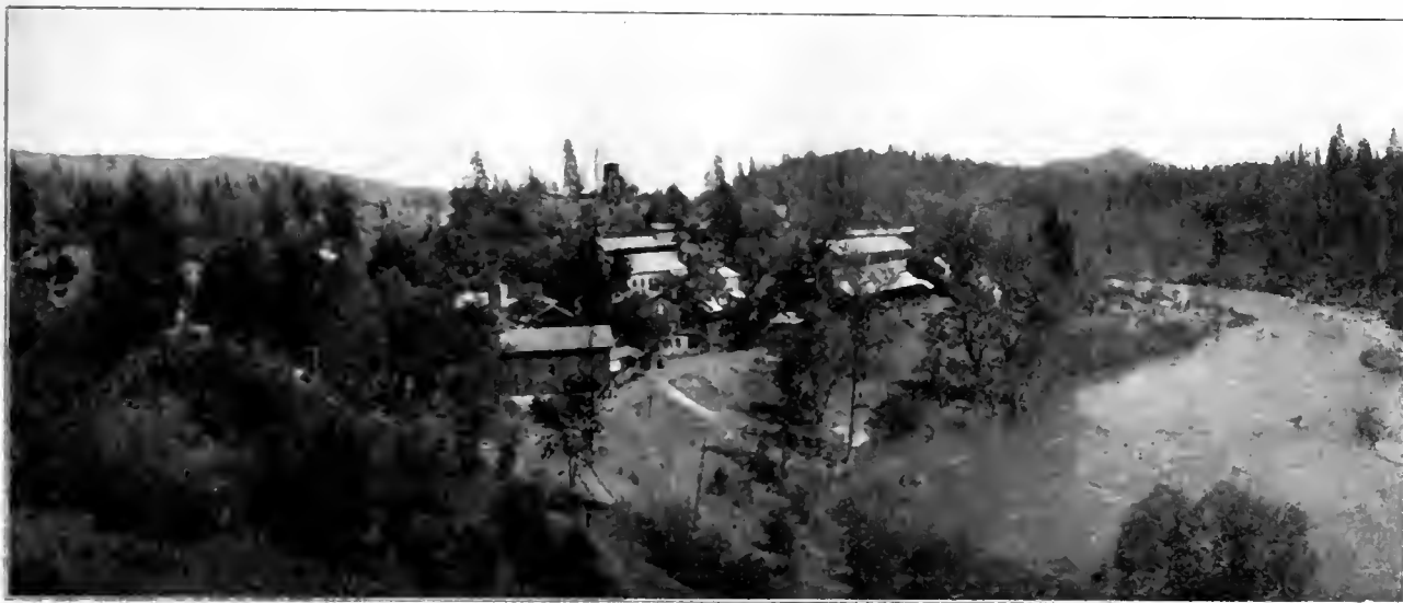
NOBLE ELECTRIC STEEL CO.'S PLANT AT HEROULT, CALIF.
