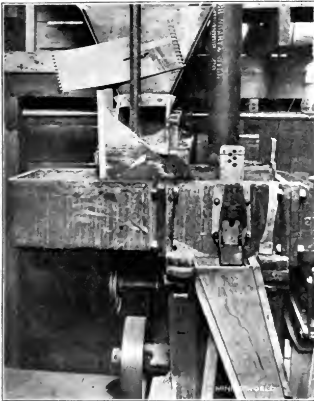
RICHARDS PULSATOR JIG IN DUNCAN MILL.
