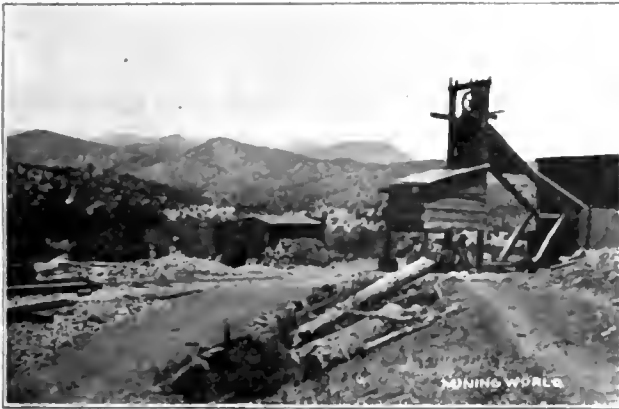
HOIST AND POWER PLANT, SILVER CELL.
