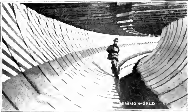
SHOWING METAL FLUME UNDER CONSTRUCTION.
