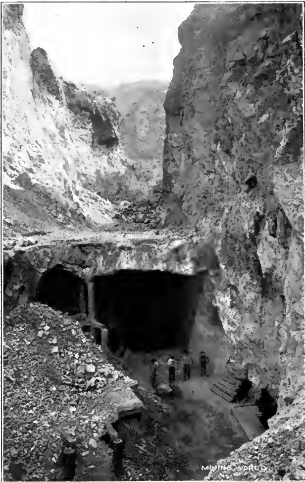
SURFACE WORKINGS OF ARIZONA COPPER CO.
