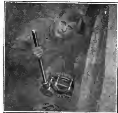
PIPE THREADING IN A TIGHT PLACE.
