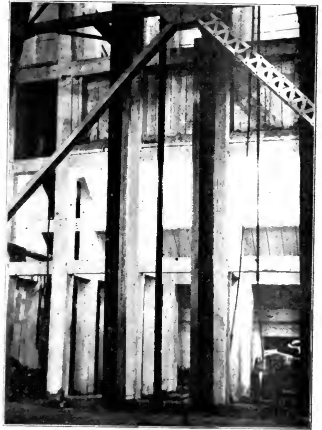
BACK VIEW OF SKIP CHUTES.
