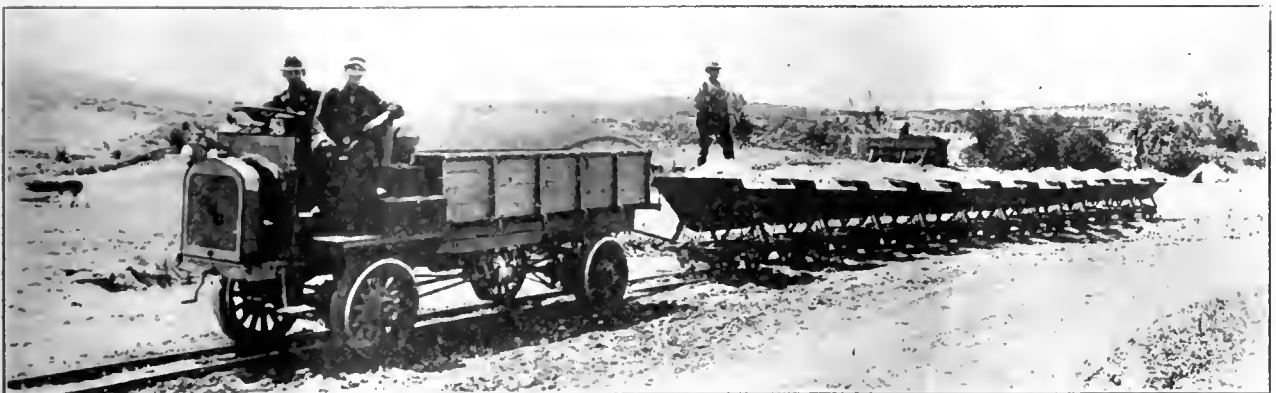
A 4-WHEEL DRIVE TRUCK HAULING GRAVEL ON A NARROW GAUGE TRACK.
