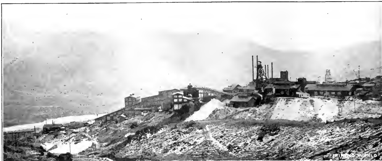
BUTTE & SUPERIOR CO.'S MILL AND FLOTATION PLANT, MONTANA.
