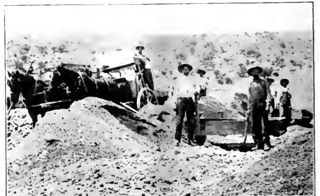
HUBBARD TUNGSTEN MINES USING MEXICAN ROCKER.
