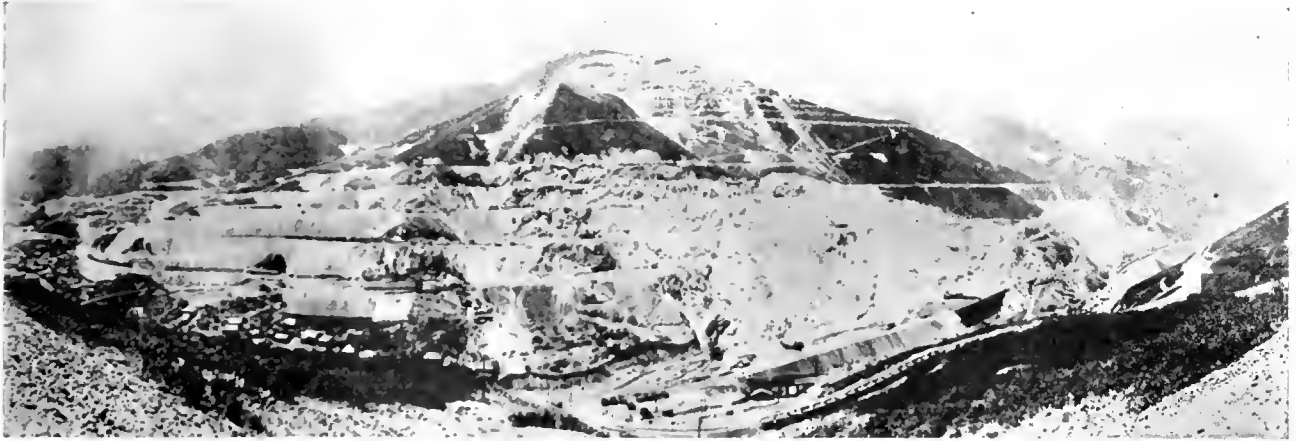
OPEN CUT WORKINGS OF UTAH COPPER PROPERTY—LARGEST COPPER DIVIDEND PAYER IN 1916.
