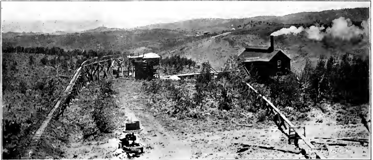
PYRITIC SMELTER OF VULCAN MINES & SMELTER CO., AT VULCAN, COLO.
