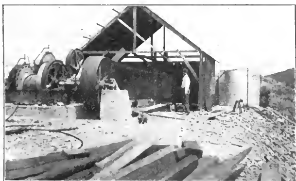
125-HP. LIDGERWOOD HOIST BEING INSTALLED.
