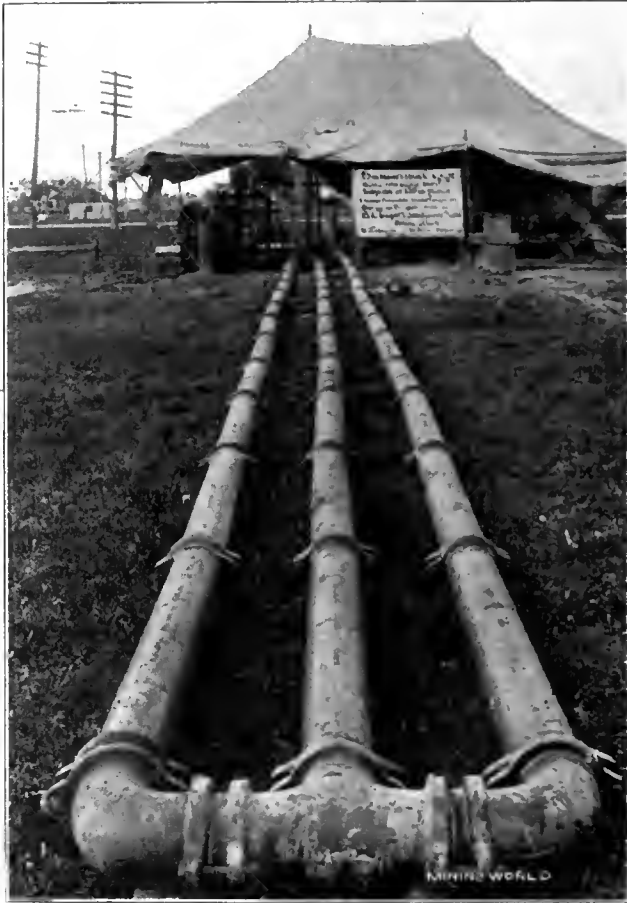
COMPRESSED AIR RESERVOIRS MADE FROM PIPE.
