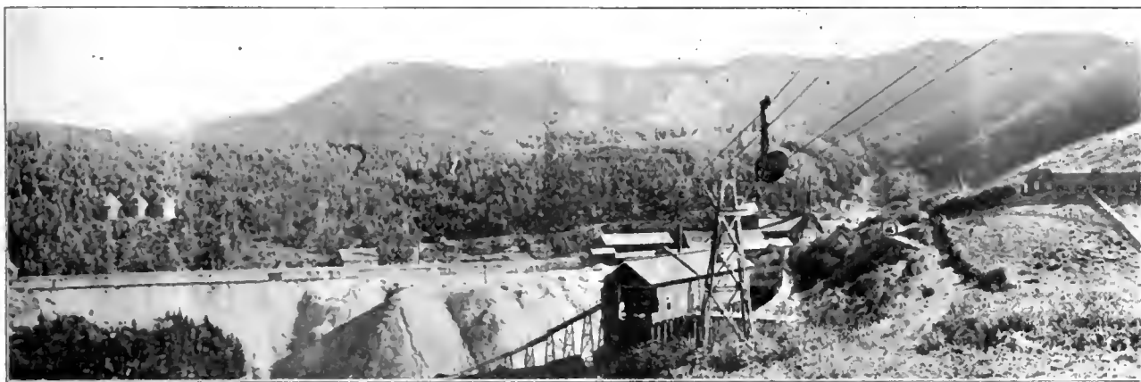
SILVER KING COALITION MINES CO., PARK CITY, UTAH. UPPER TERMINAL OF TRAMWAY IN FOREGROUND.
