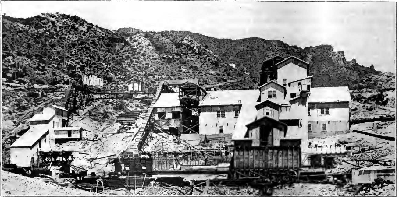
MILL AND SURFACE PLANT OF MAGMA COPPER CO., ARIZONA.
