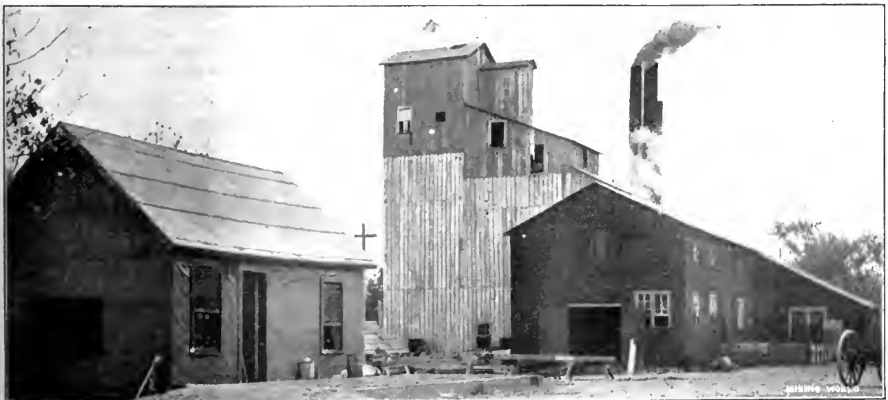
SURFACE PLANT OF PITTSBURGH MINE, WISCONSIN.
