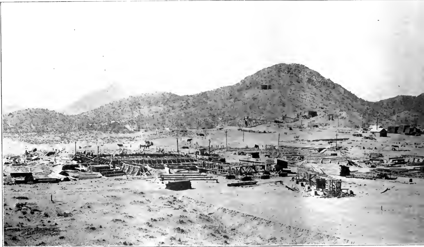
Foundations for Power House and Electrolytic Plant.
