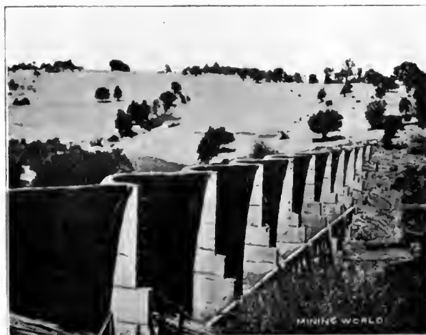
THE ARGONAUT TAILINGS DAM.
