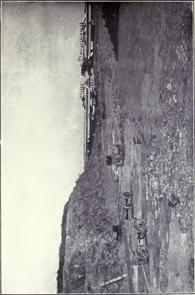
Fig. 53.—Mining Bank of Shale by Hand.
