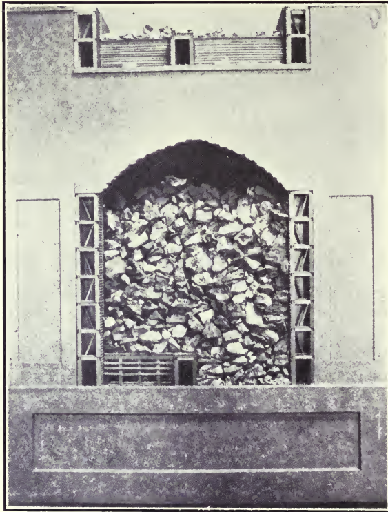
Fig. 37.—End View of Stope in Homestake Mine, Back-filling Method. From Model in Engineering Office of Company.
