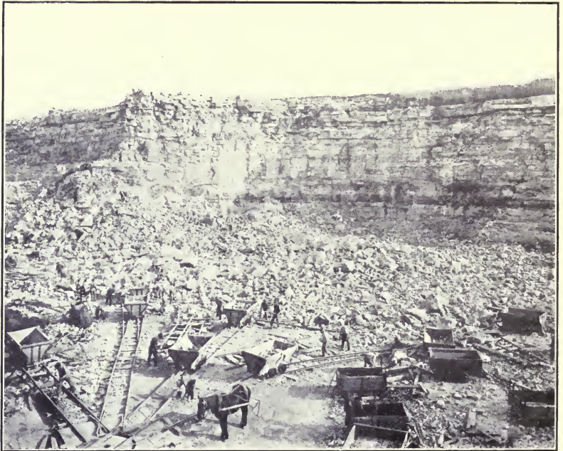
Fig. 55.—Quarry showing Result of Blast.
