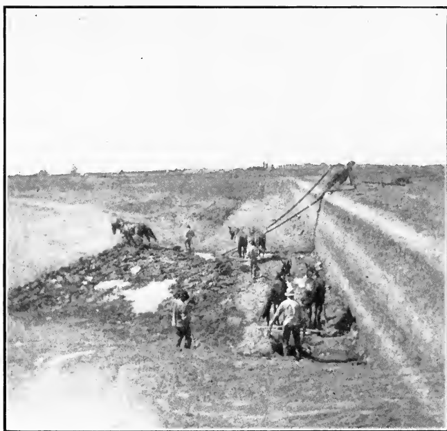
Fig. 56.—Stripping Coal by Scrapers.
