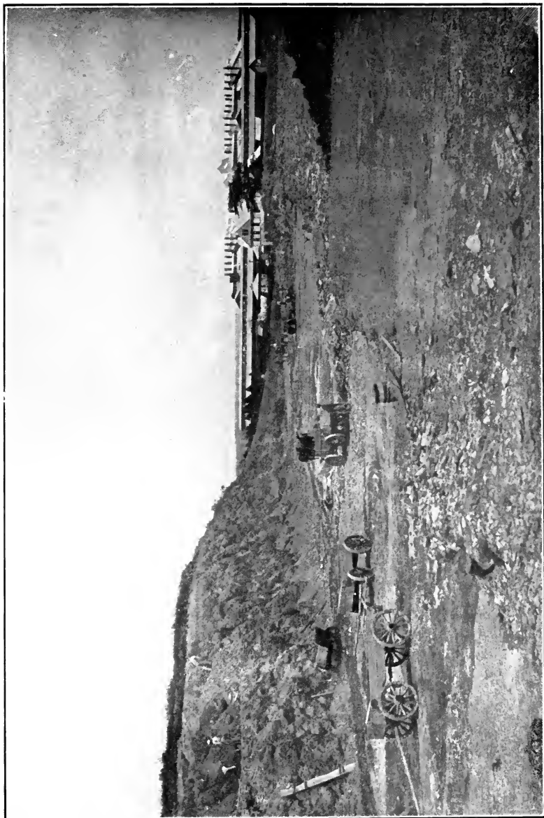
Fig. 53.—Mining Bank of Shale by Hand.
