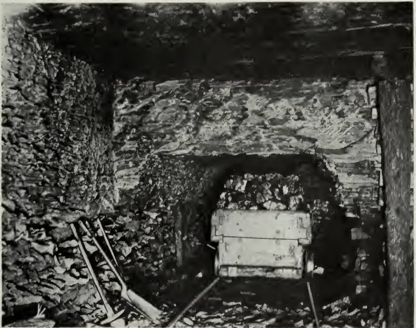
FIG. 20. Amount of "company brushing" necessary after subsidence
