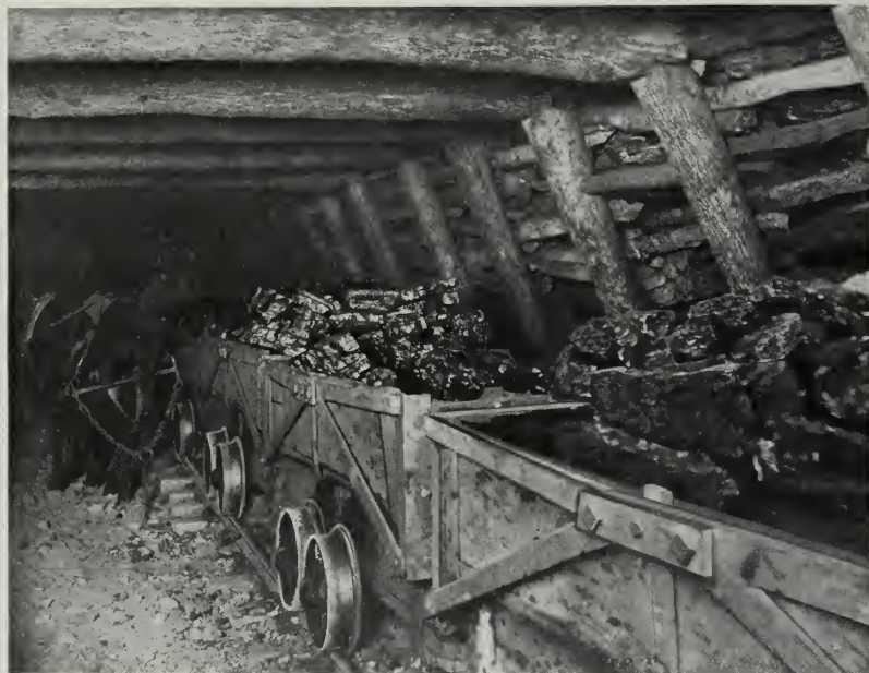
FIG. 15. An entry closely timbered. (Photo by J. J. Rutledge)
