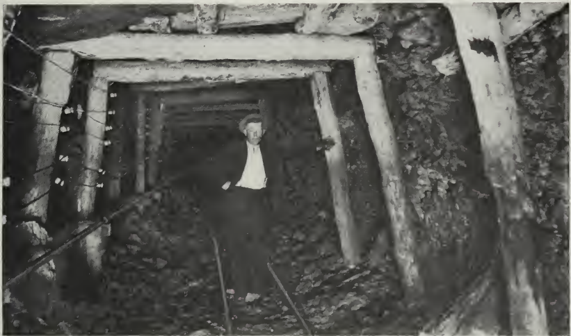
FIG. 6. Entry in mine with no shaft pillar
