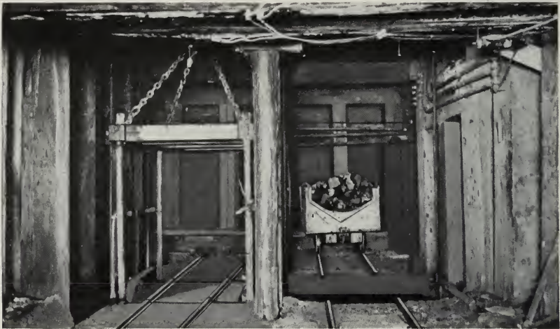
FIG. 21. Typical shaft bottom
