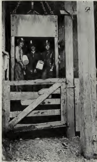
FIG. 23. Skip adjusted to hoist men
