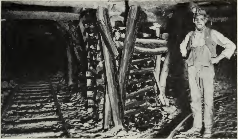
FIG. 16. Cog built of props
