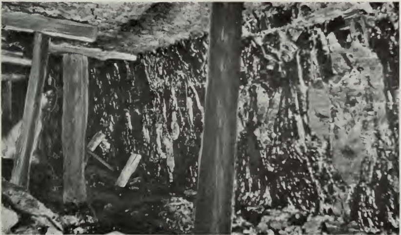
FIG. 13. Props at working face
