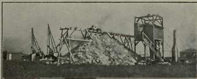
FIG. 12. DRILLING AND SHAFT SINKING NEAR PICHER, OKLA.
