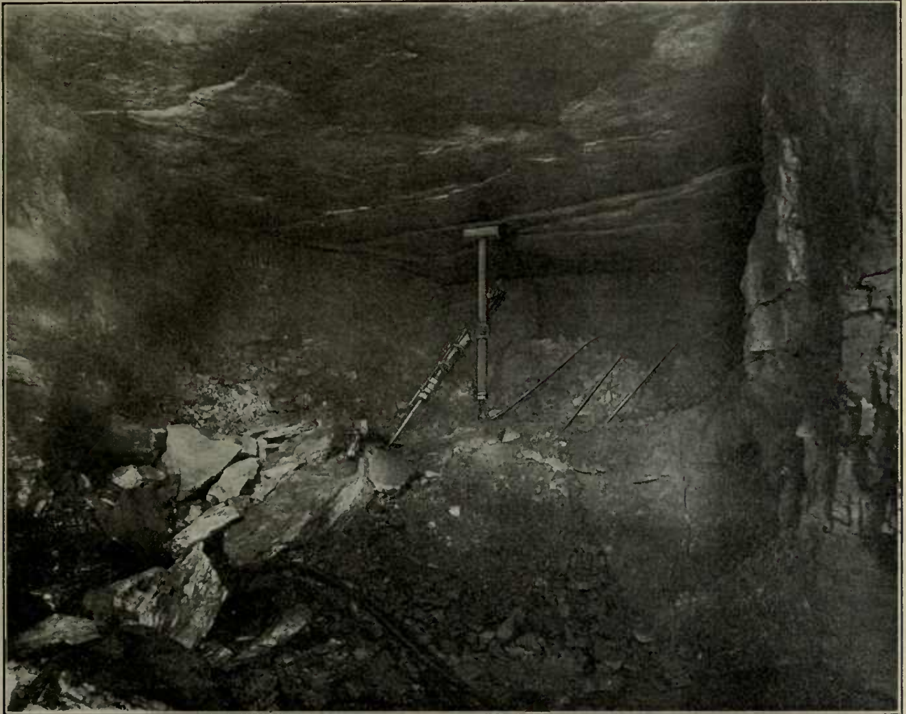
FIG. 18. STOPE HEADINGS ARE ADVANCED DRILL COLUMN HIGH CLOSE TO THE BACK, AND ORE BELOW THE HEADING, IF ANY, IS UNDERSTOPED IN BENCHES PROGRESSIVELY, LEAVING COLUMNAR PILLARS IN THE OREBODY, SPACED AND PROPORTIONED ACCORDING TO HEIGHT AND STRENGTH OF THE ROOF OR GRADE OF THE ORE
