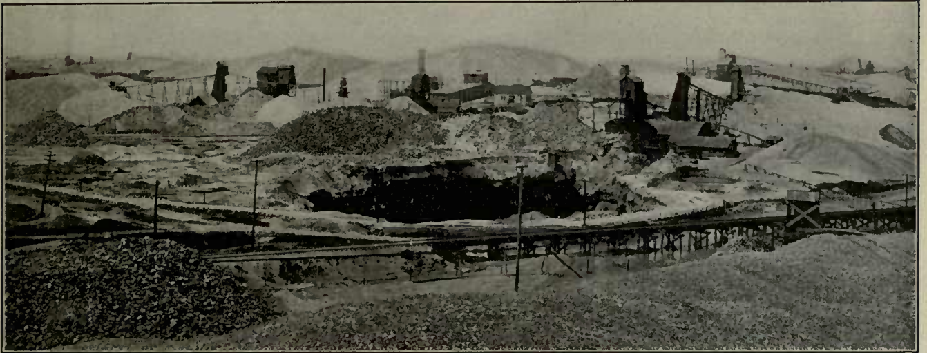
FIG. 6. TYPICAL VIEW IN THE SHEET-GROUND AREA, SHOWING EFFECT OF A CAVE
