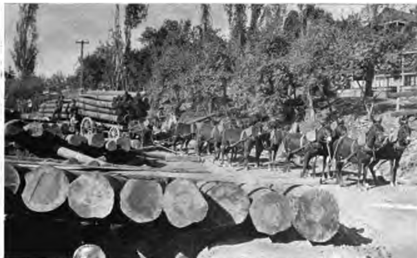
TIMBER FOR UTICA MINE.
