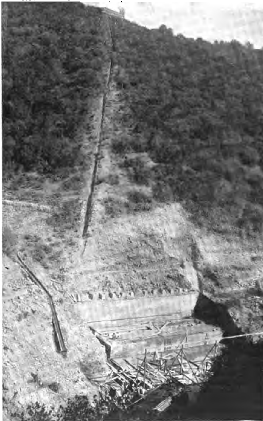
FOUNDATION AND WATER POWER OF GWIN 40-STAMP MILL.
