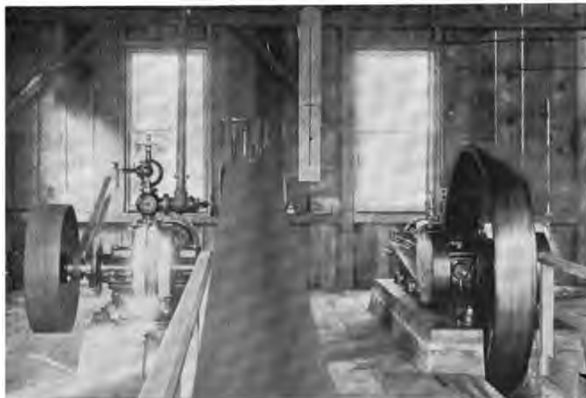
THE HOIST AT THE MELONES.
