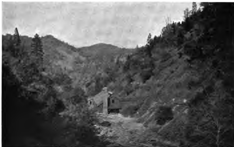
THE ESPERANZA CHLORINATION WORKS.
