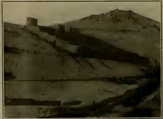
NEW MILL, BRADEN COPPER CO.
