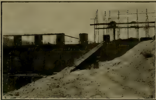
MIAMI MILL WHILE UNDER CONSTRUCTION.
