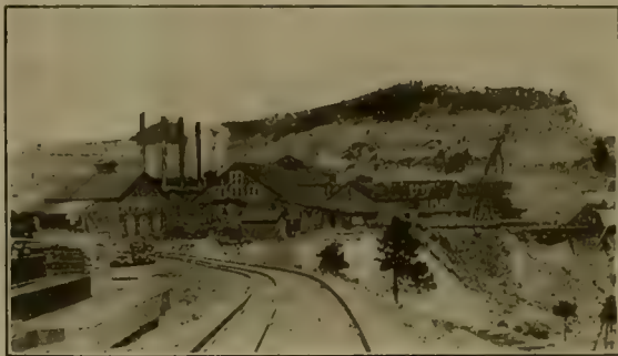
HIGHLAND HOIST, HOMESTAKE MINE.
