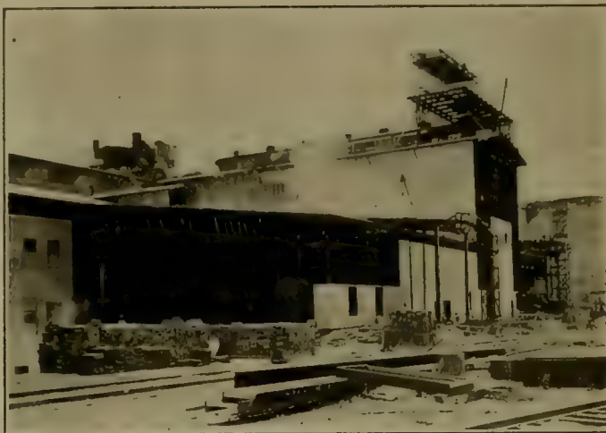
KILNS OF RIVERSIDE PORTLAND CEMENT CO., SHOWING EXPERIMENTAL COTTRELL UNIT AT LEFT AND ERECTION OF PERMANENT EQUIPMENT AT RIGHT.
