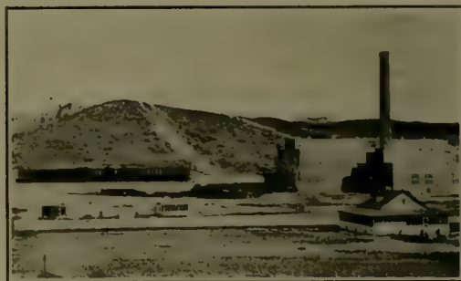
POWER-HOUSE AT MIAMI.
