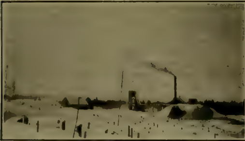
HOLLINGER NO. 1 SHAFT AND TEST MILL.
