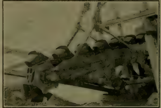
CONREY NO. 2 IN WINTER, BEFORE THE 14-FT. OPEN-CONNECTED CHAIN WAS CHANGED TO 9-FT. CLOSE-CONNECTED.
