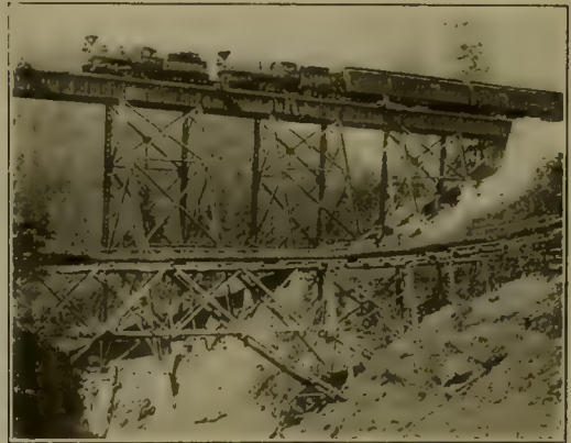
INEXPENSIVE PIPE TRESTLE.
