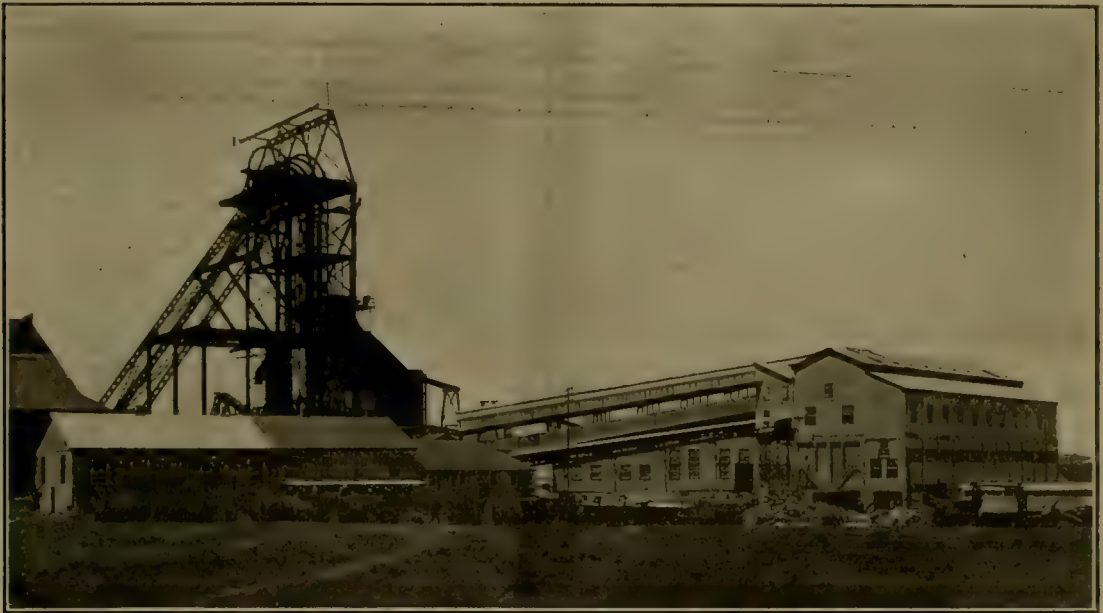
THE CITY DEEP SHAFT, JOHANNESBURG.
