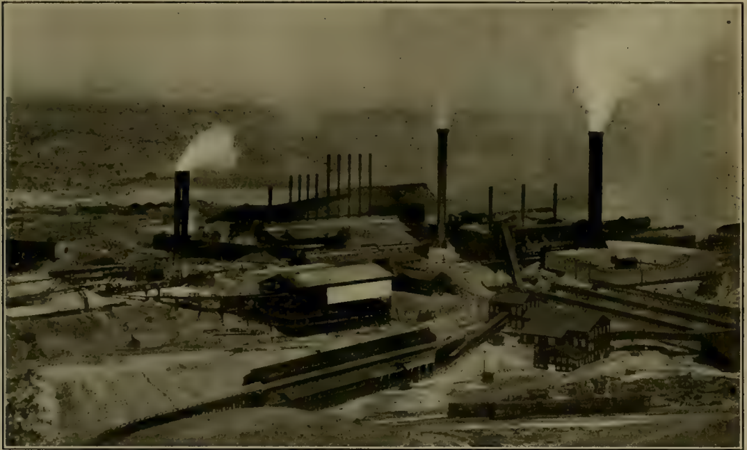
FIG. 1. GENERAL VIEW OF SMELTING PLANT, GREENE-CANANEA COPPER CO.
