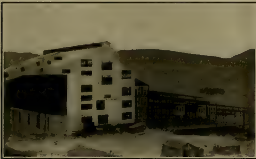
RAY CONCENTRATOR, FROM TOP OF POWER-HOUSE.
