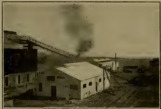
CHINO MILL, WHILE UNDER CONSTRUCTION.
