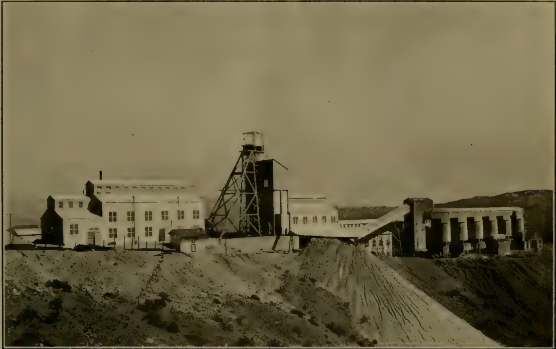
MAIN HOISTING SHAFT AND ORE-BINS, MIAMI COPPER COMPANY.
