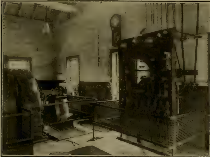
SAFETY DEVICES AROUND MACHINERY AT MINES OF OLIVER IRON MINING COMPANY.
