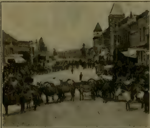
PACKING CABLE FOR THE NELLIE TRAMWAY, TELLURIDE.
