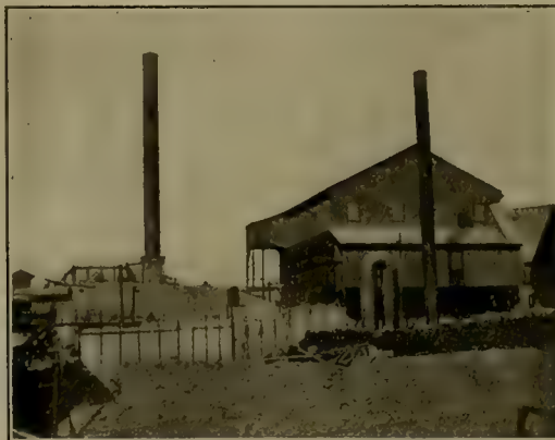
THIOGEN PROCESS PLANT, CAMPO SECO.
