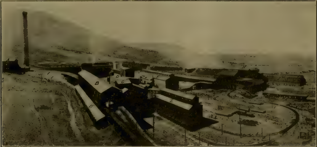
COPPER SMELTING PLANT, INTERNATIONAL S. & R. CO.
