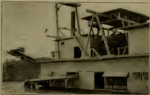
DREDGING AT OROVILLE.
