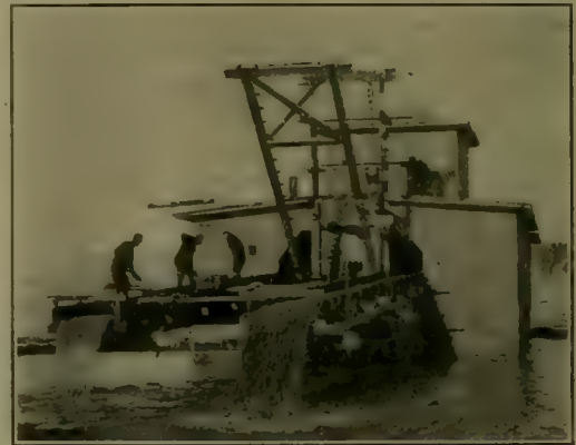
TIN-DREDGE, SHOWING ONE SLUICE BEING CLEANED UP.
