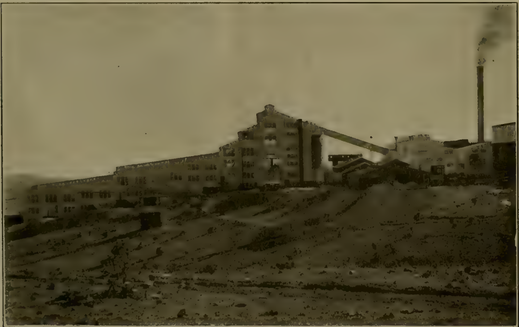
CHINO POWER-PLANT, MILL, AND MACHINE SHOPS, HURLEY, NEW MEXICO.
