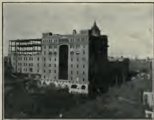
'Corner House' Central Administration Bdg, Johannesburg.
