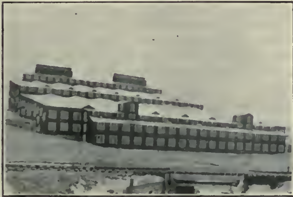
Main Mill Building.
