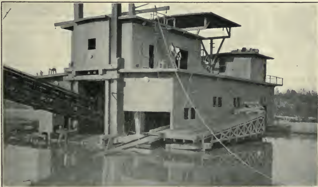
Shasta Dredge on Clear Creek.
