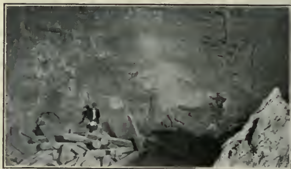
Fig. 2. Caved Square-Set Slope, Arizona Copper Co., Morenci.
