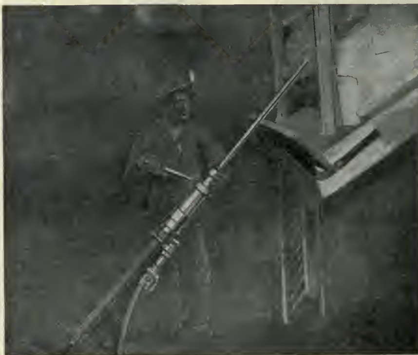
Sullivan Hammer-Drill Block-Holing.
