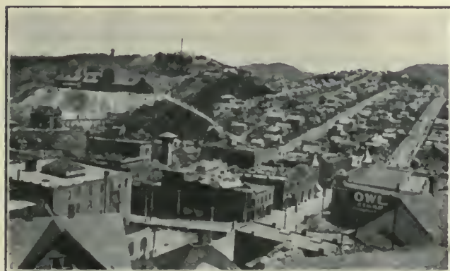
Lead, S. D., Elison Hoist in Foreground, Water Reservoir on Hill.
