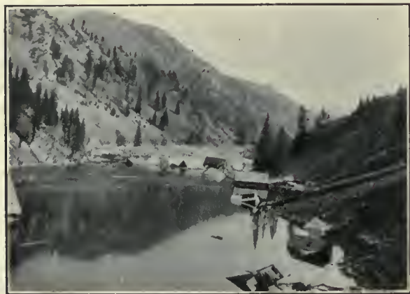
Town of Roosevelt, Looking Down Stream Toward the Mud Dam
