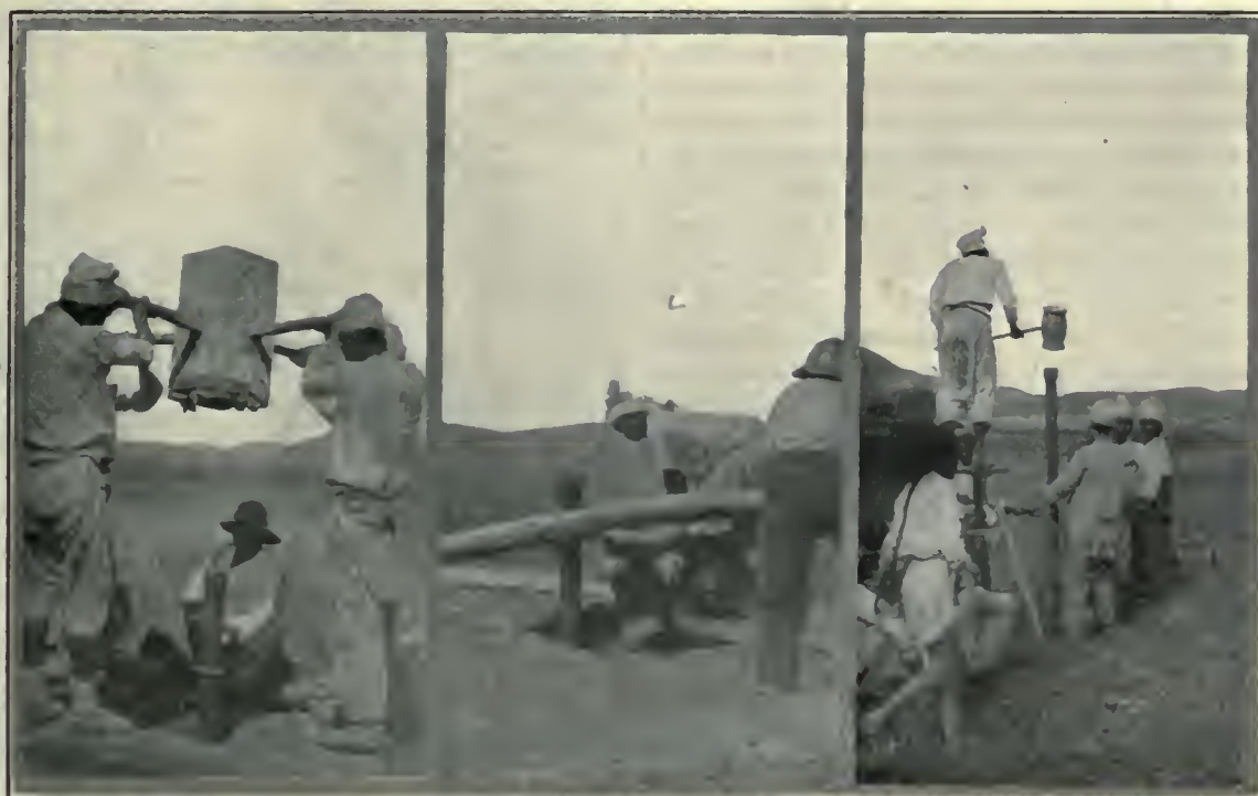
Drilling in Alluvial Ground in Korea.
