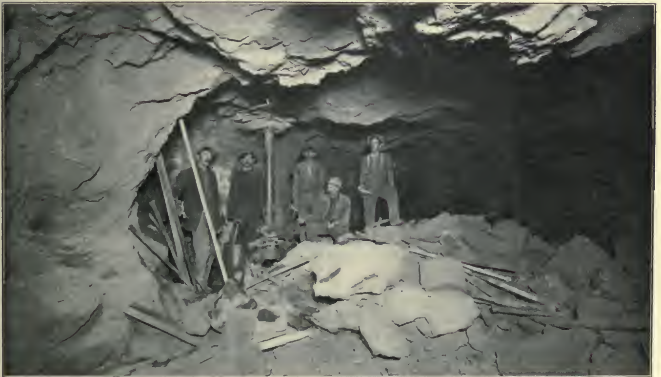
Stoping in Mason Valley Mine.
