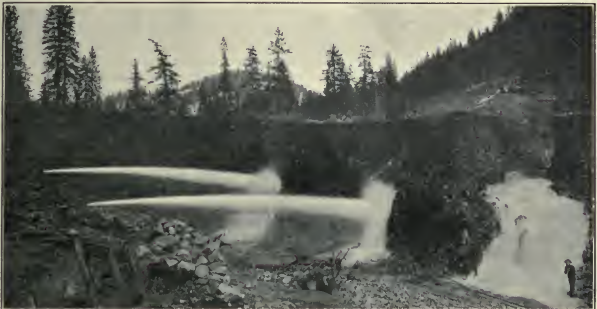
Use of By-Water With Giants in Hydraulic Mining.
