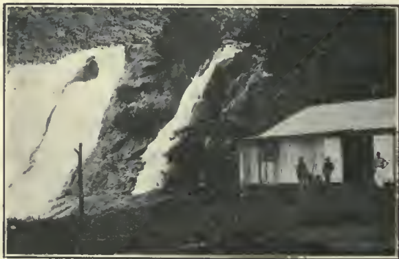
Siempre Viva Falls and Power Station.
