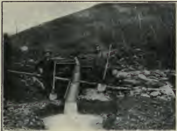
Sluicing on Dahl Creek.
