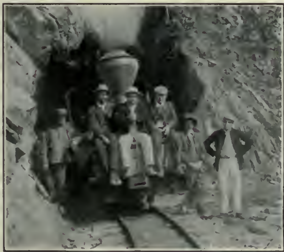
Tunnel on Pakadong Railroad.
