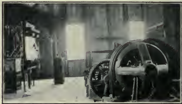
Fig. 3. Interior Showing Hoist, Switchboard, and Light Construction of Building.
