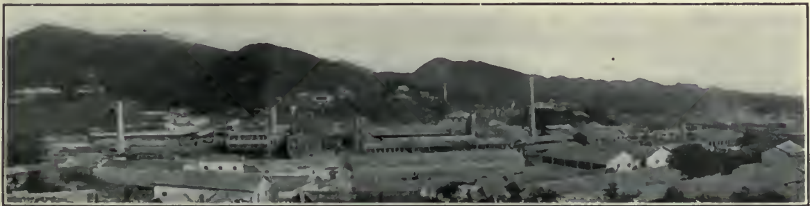
Pinghsiang Colliery, General View.
