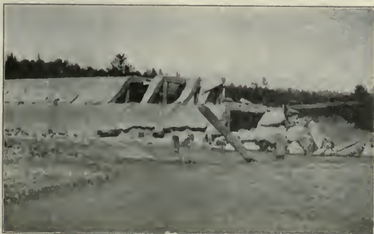
Fig. 4. Near View of North End of Break.
