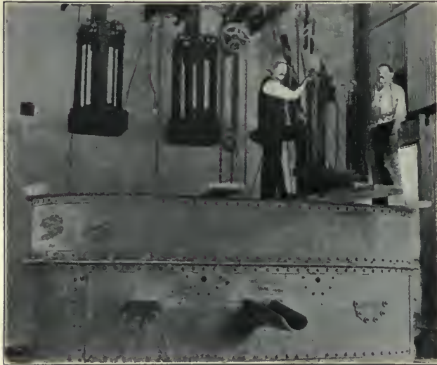
Heroult Smelter in Course of Construction.
