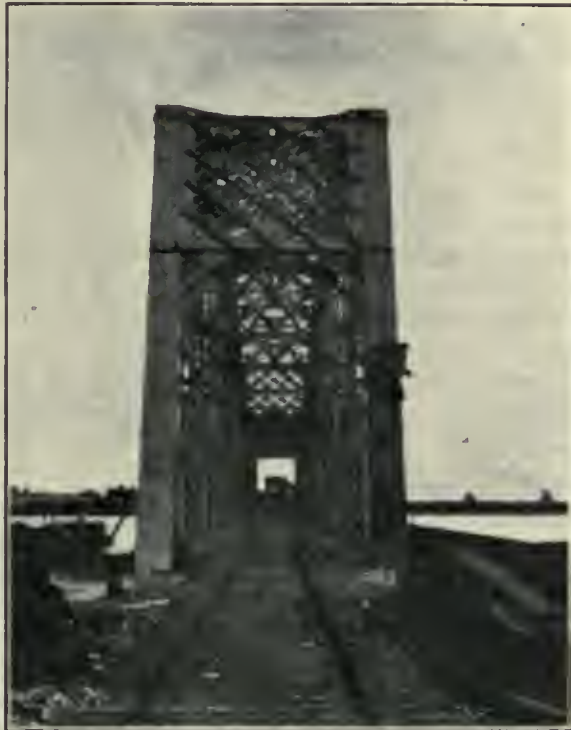
Flag Point Bridge on the Copper River & North-Western Railroad.
