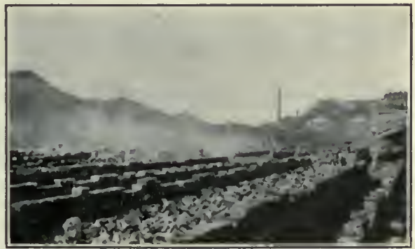
Coke Ovens at Pinghsiang Colliery.
