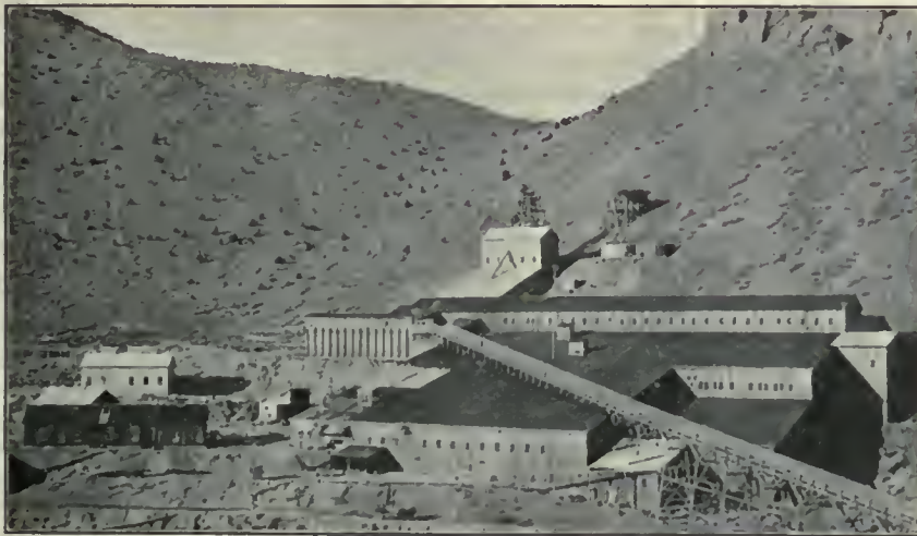
Butters Cyanide Plant, Six Mile Canyon.
