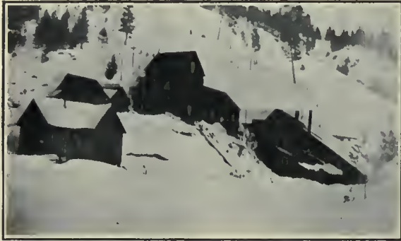
Pioneer Shaft, Gold Hill Mine, Quartzburg, Idaho.
