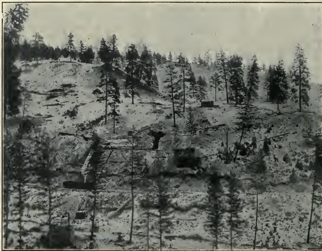
Part of Surprise Mine, Republic, Washington.
