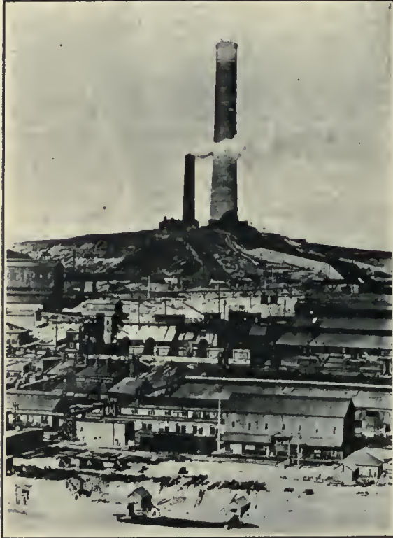
Great Falls Smelter and Chimney.
