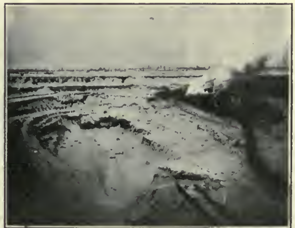
Stripping and Mining at the Same Time. Shenango Mine.
