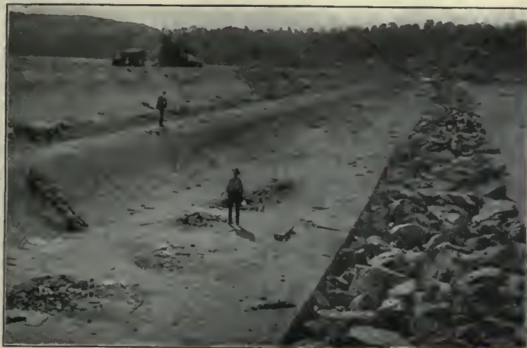
Fig. 2. Yuba River Barrier, on October 4, 1905.
