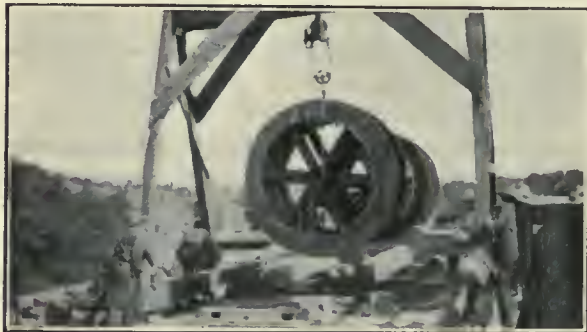
Fig. 2. Crane Carrying Ore-Hoist Drum Weighing 6000 Pounds.
