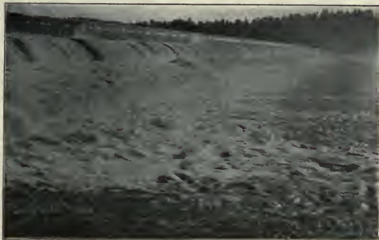
Fig. 3. Yuba River Barrier After Freshet of January, 1906. Water 1.4 ft. Deep on Crest.
