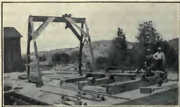
Fig. 1. Crane and Bed-Plate of Hoist.
